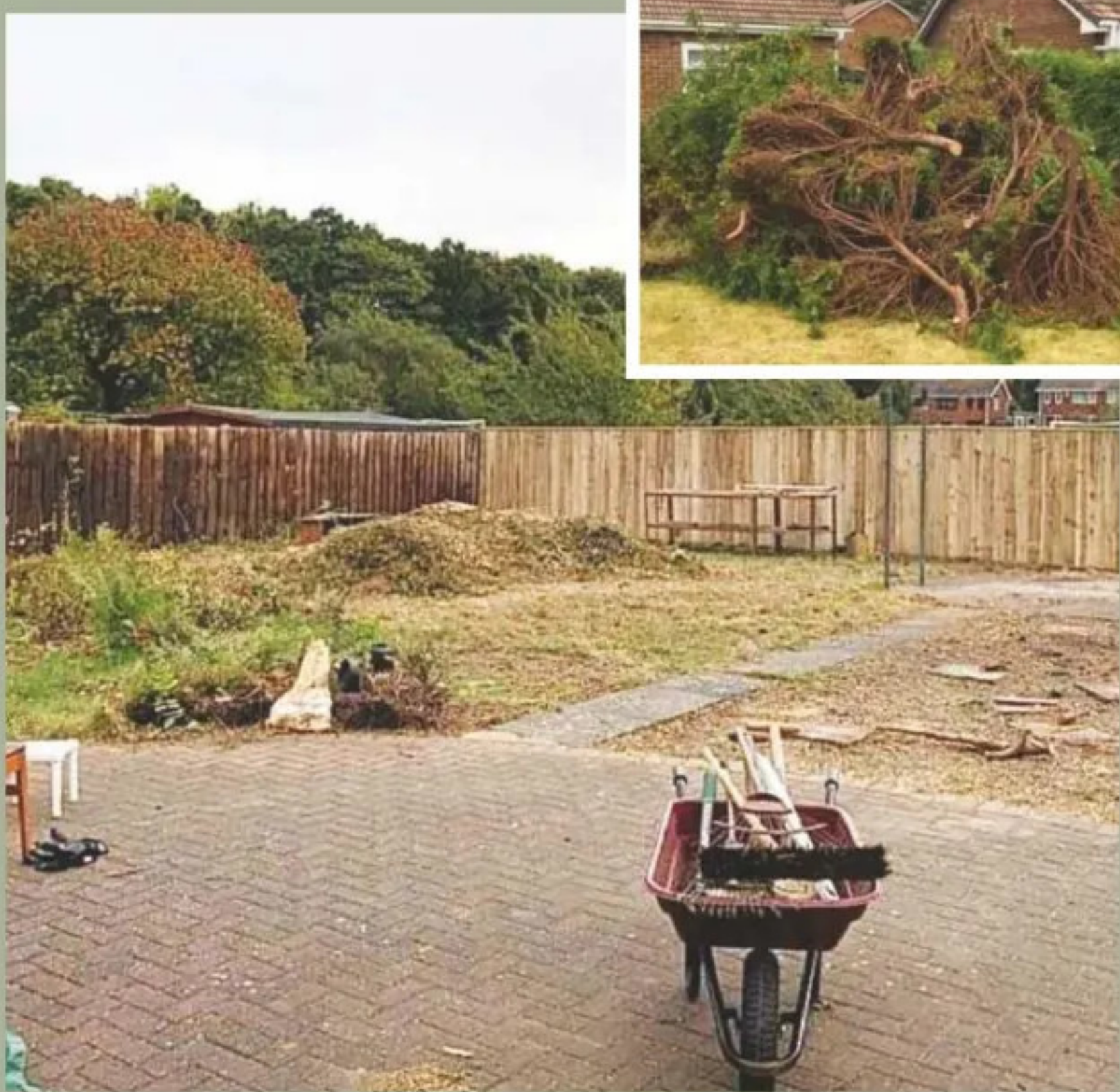
2 With the hedge taken out, we were amazed at how much extra garden was revealed. In fact, this space was increased by an extraordinary 4m in width and 2m in length. I helped to remove some of the larger section trunks. Carl had already cut down the foliage and small section trunks, as well as hiring a chipper/mulcher to reduce all branchwood and smaller pieces to chips; these could then be used as mulch in the garden, so nothing was wasted
