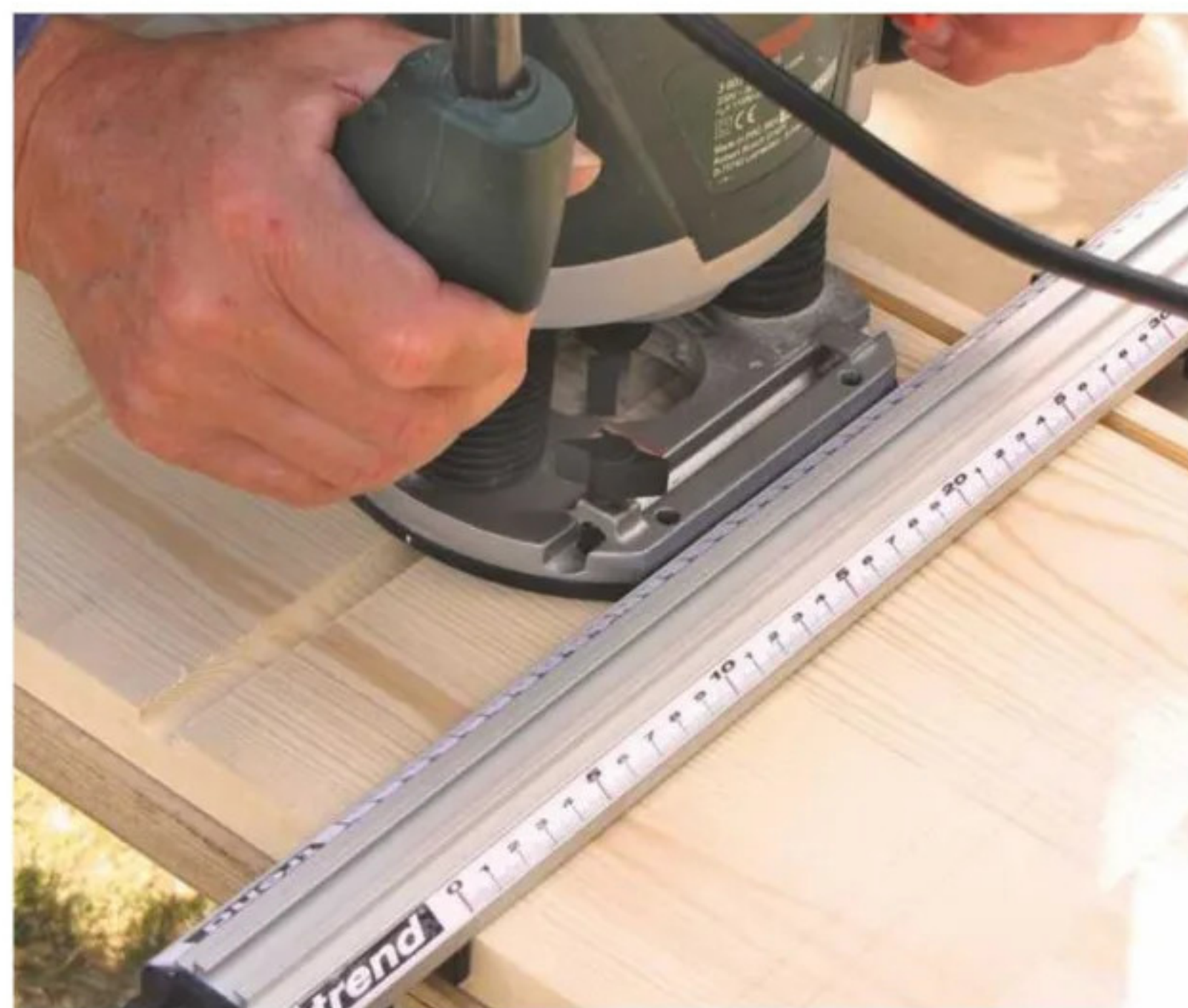
11 Using a 12mm cutter, rout housings for the divider panels across top and bottom pieces
