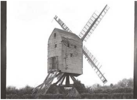
3 Post mill in Ashurst, Kent...
