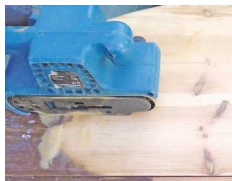
14 Initial clean-up of table top with a belt sander
