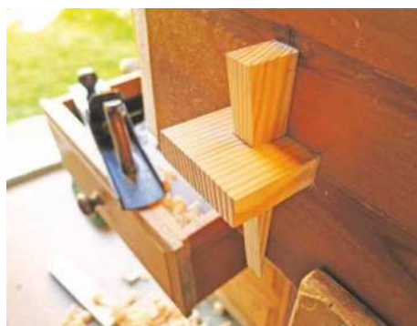
13 Peg inserted before shaping
