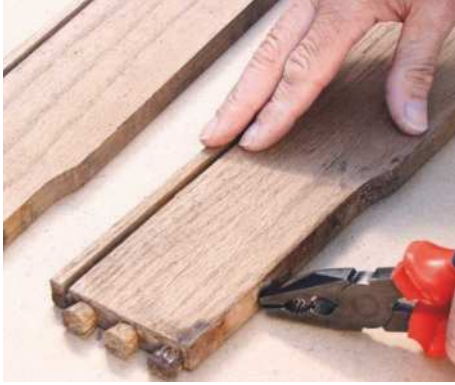
1 When recycling timber always remove old screws and nails first. If rusted, plan saw cuts to avoid defects
