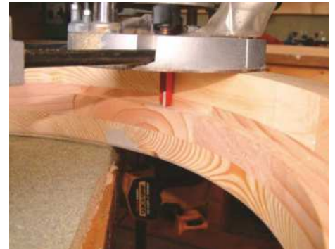
11 Mark the frame position, remove and mount upside down. Rout the rebate for the glass
