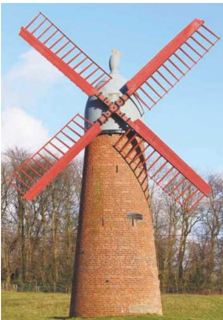
6 Tower mill in Haigh, Greater Manchester
