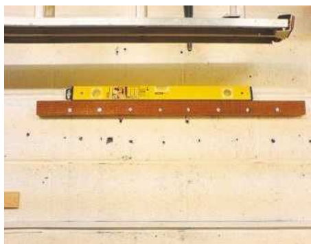
20 Attach one of the cleats to the wall, ensuring that it's level
