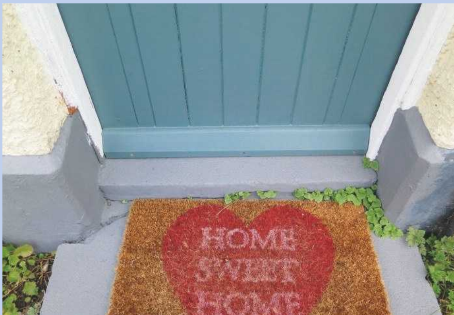
11 Weatherboard fitted and sealed to the door with silicone
