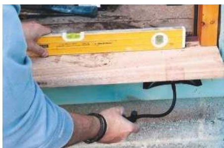
It's equally simple to lift the frame as a unit or adjust one side for level
