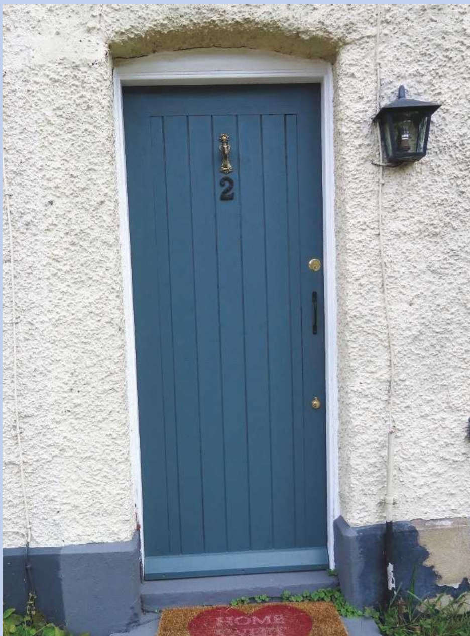
13 New door looking smart having received several coats of paint
