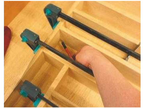
12 Mark out all intersections ready for the biscuit slots to be cut
