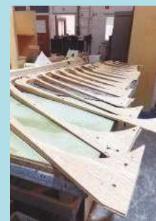
Tapered pieces ready for laminating
