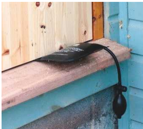
Doors can be wedged but over-inflation with minimal insertion can make them slip out
