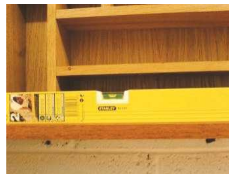
21 Once the other cleat has been attached, lift the cabinet onto the wall
