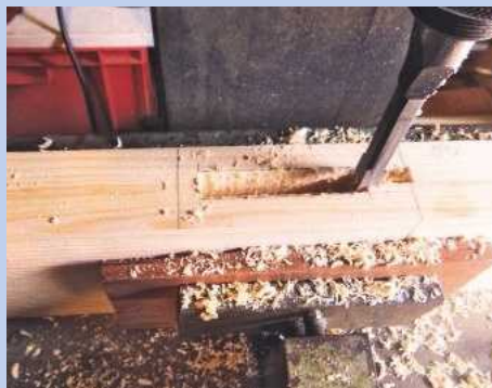
6 Cutting 15mm mortises with a 10mm chisel
