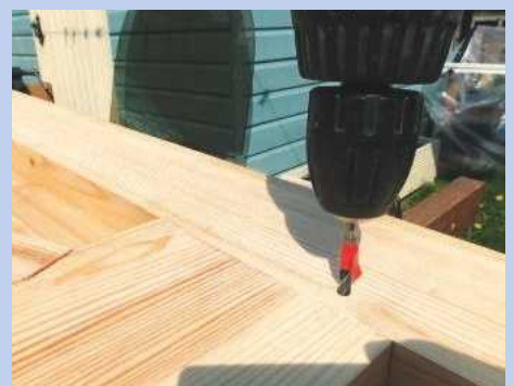
10 Drilling 6mm holes for the dowels
