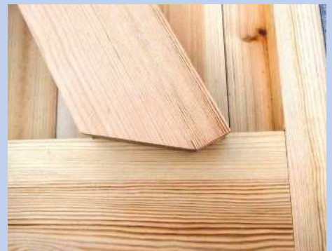
7 Diagonal brace before marking and cutting into the rail
