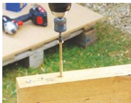
I managed to drive 6.0 x 100mm screws into softwood and oak without pilot holes
