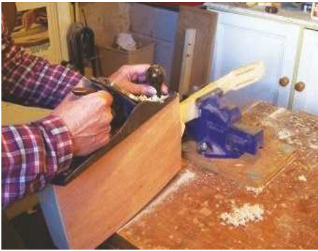
37 Planing back edges flush with the sides
