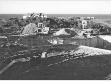
At the house site, the massive concrete coffer dam foundations went down...
