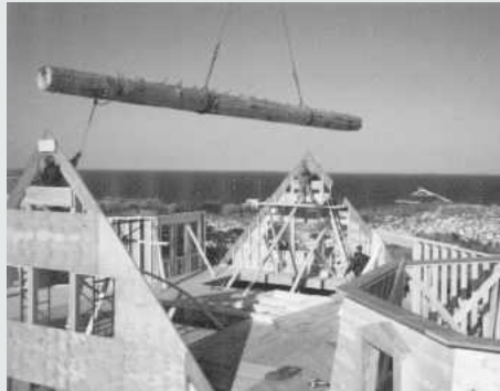
... and slowly lowered inch by inch towards the huge gable end walls of the main house
