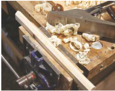
14 Plane the ridge piece's top edge to a point
