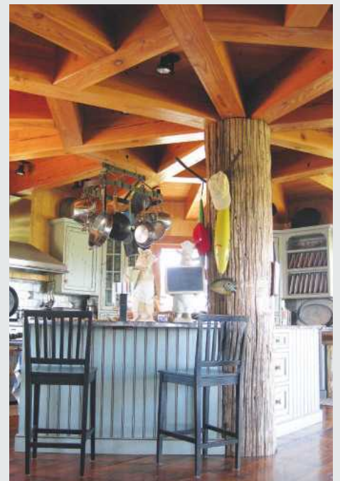
A spare beam supports the joists for the floor above the kitchen
