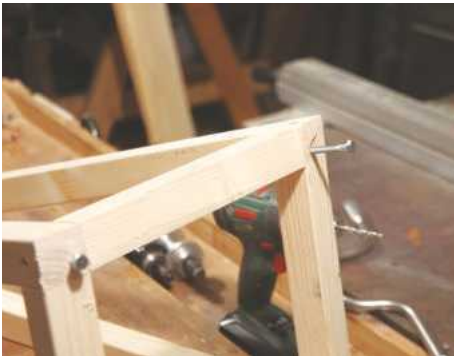
4 Fit coach screws to the base of each post
