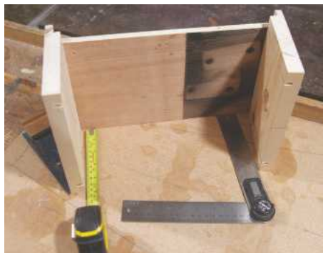
8 Ensure the tops of the ends are all level
