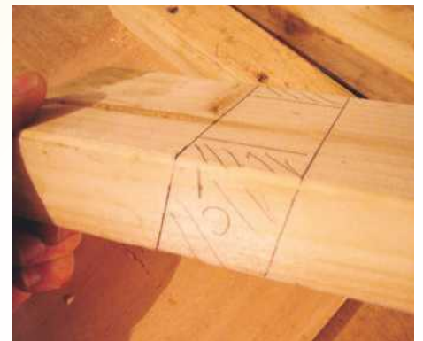
4 All marked out and ready to cut the first housing. Remember to label clearly
