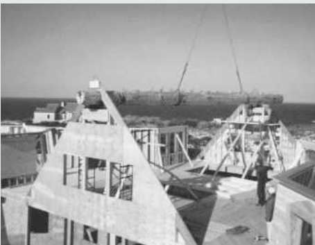
Each end had to be fitted into a circular cutout in the timber-framed gable
