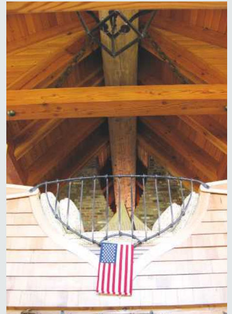
The Beam is currently playing both a starring and a – roof – supporting role
