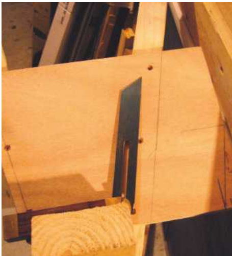
8 Check with the bevel and squeeze, if necessary, before starting to screw leg to ply gusset
