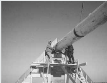
With one end in position, the other was skilfully threaded into its cutout
