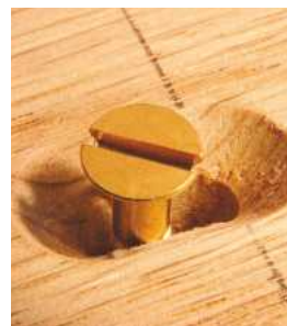
27 On the underside of a solid wood cabinet top, glue is avoided and instead screws in slotted holes allow for seasonal movement
