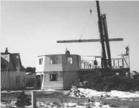
The log – soon to be The Great Beam – was carefully craned into the sky...
