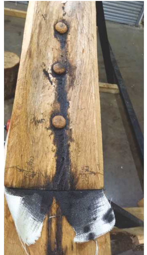
Joint between stern underlute and stern-post treenails and caulking
