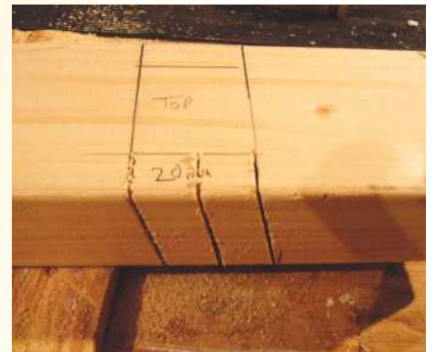
2 Cut to the line, including a central cut to make waste removal easier; clean up with a chisel
