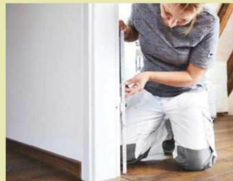
2 Measure the distance along the frame from the top edge of the door hinge to the floor
