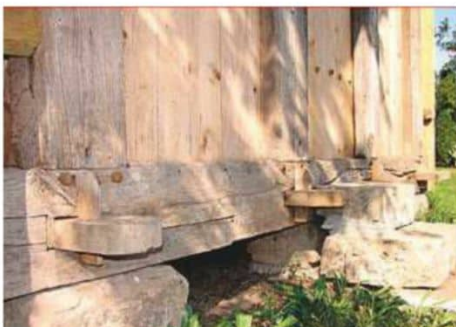
Tusked through tenons used on a French granary
