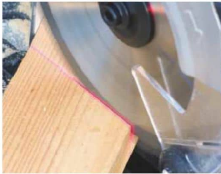
The laser line extends over the front edge of the timber, which helps in lining up the blade with your pencil mark
