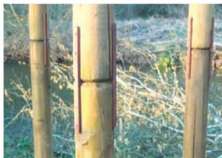
1 Stilt poles extended by routing in steel locating pins and brackets
