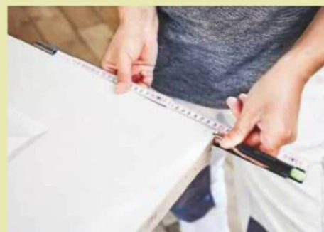
3 Lay the door on two stands, which will ensure you're able to work in a comfortable position. Transfer the measurement you've just taken
