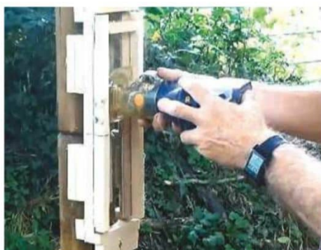
2 An improvised jig for cutting grooves, using a Ryobi cordless router
