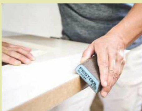
7 The cutting edges should be ground if required, ideally using a hand-sanding block or abrasive sponge
