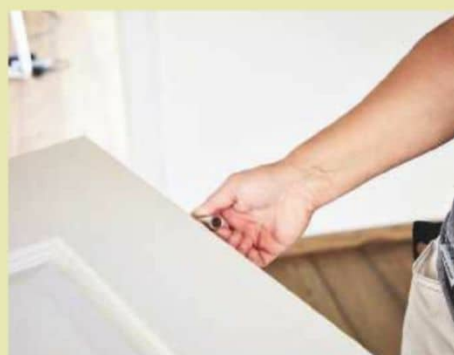
8 You won't know if you've been successful until the door is hung. Any fine adjustments can be made via the hinges
