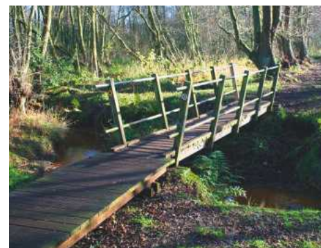
15 Wooden bridge in woodland
