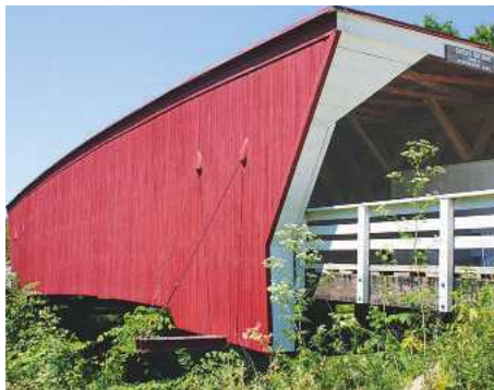
4 The Cedar Covered Bridge in 2016
