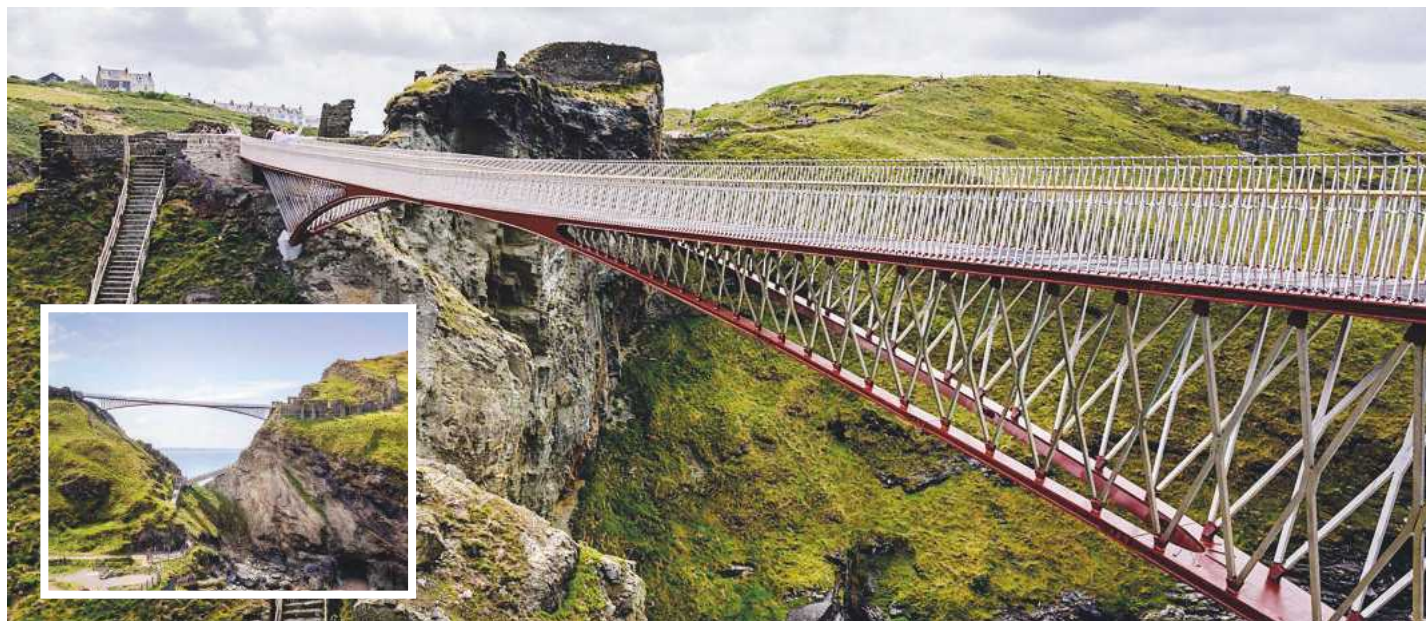
12 Tintagel Castle footbridge, built using technology usually found in the Alps, follows the path of an old land bridge
