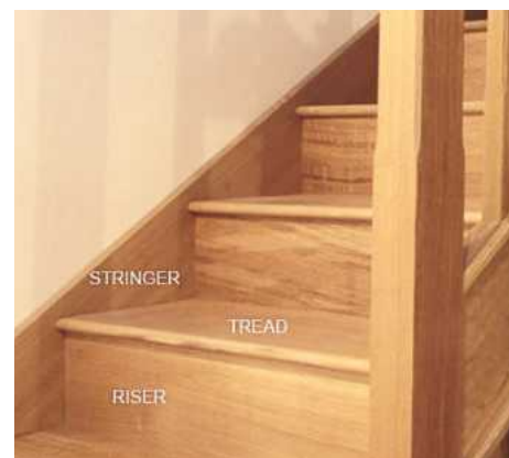
Stair stringer, tread and riser, shown here in American white oak
