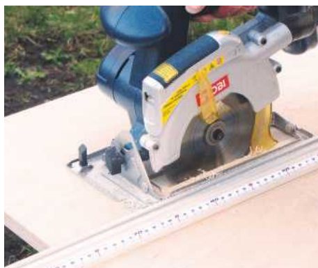
1 Start by sawing the ply to size using a guide rail. The top board is about 90mm narrower than the lower one
