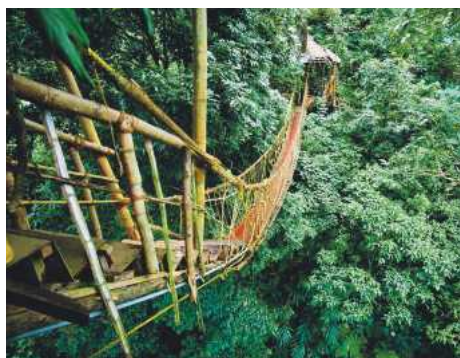
13 Hanging bridge at the tree house resort in India Photograph © Getty Images
