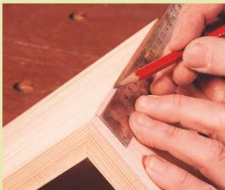
2 Mark out dovetail spacings across the joint, keeping outside splines away from the edge. Start by marking a line about 10mm in from each edge for the outside pair, then divide the space between these lines equally across the joint
