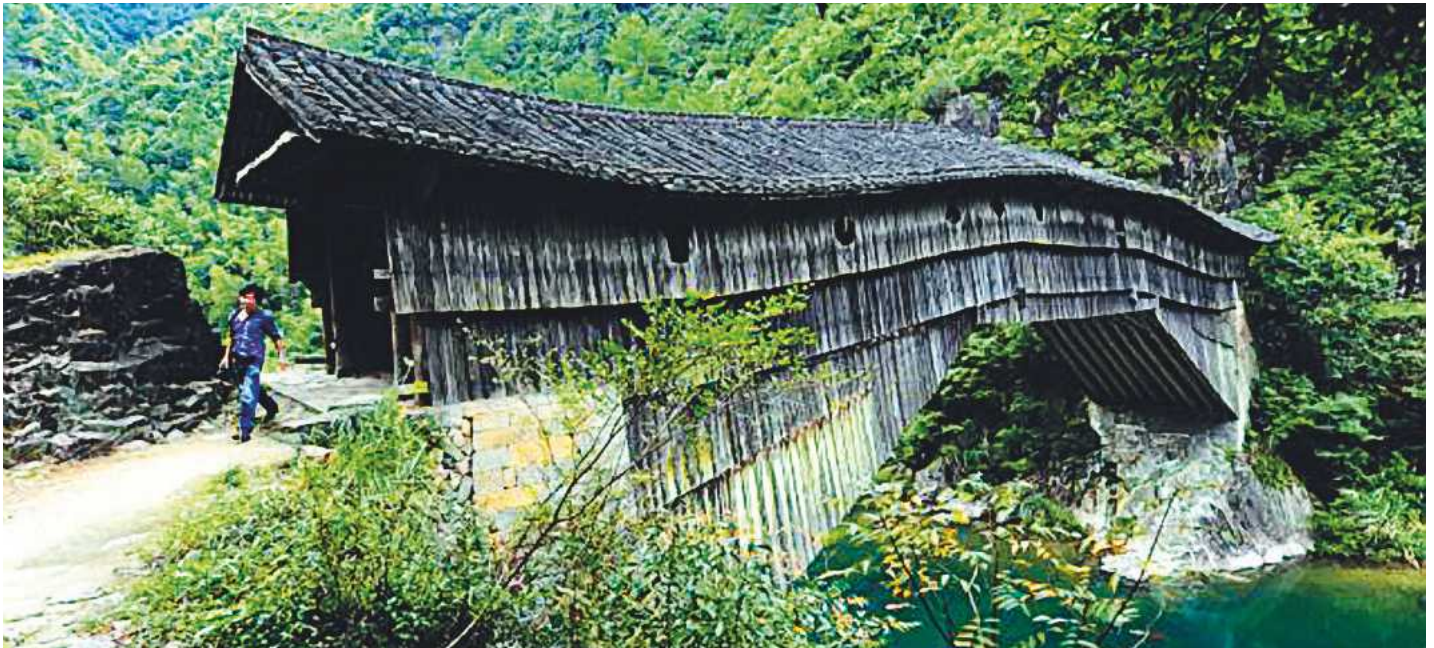
16 Yangmeizhou timber arch lounge bridge, in the Kengdi village of Shouning County, which was built during the Ming Dynasty
