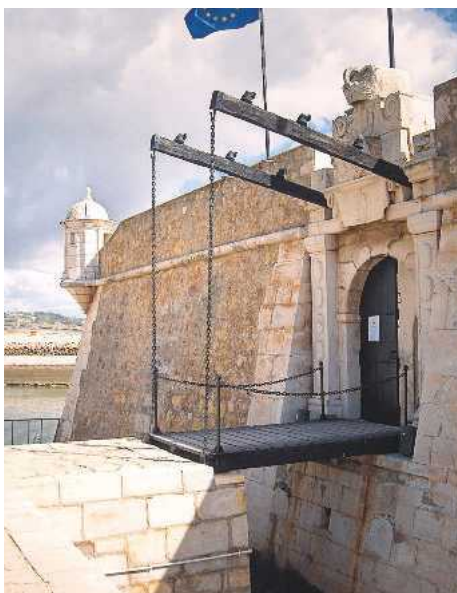
8 Drawbridge at the fort of Ponta da Bandeira, Lagos, Portugal
