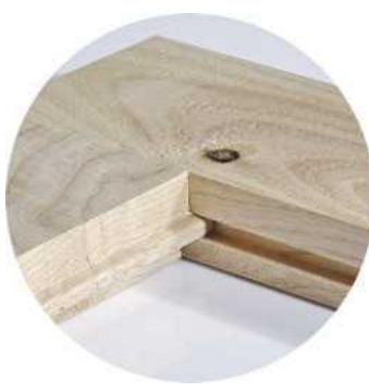
Secret nailing in parquet flooring
