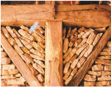
The scarf joint used on the beams above the post is known by its French name 'trait de jupiter' or 'bolt-o-lightning' joint
