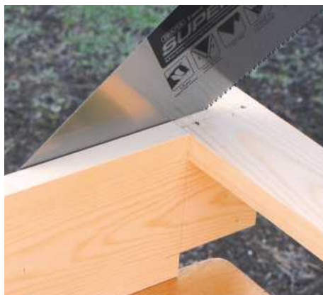
14 Saw off the horns so they are slightly proud of the sides; this will allow you to trim them flush
