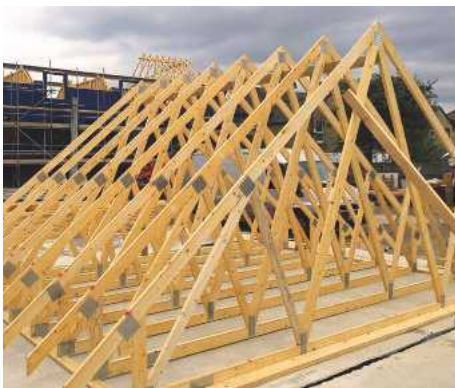
A selection of roof trusses
