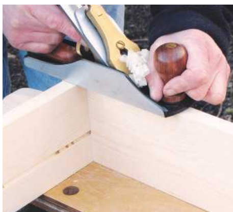
19 Carefully true up the front edges of the carcass, checking with a straightedge
