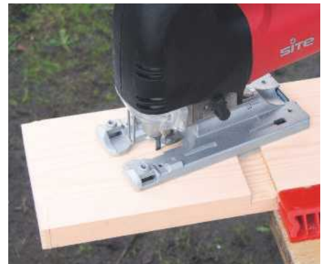
6 Fit your jigsaw with a suitable narrow blade and cut the profile, just outside the pencil line
