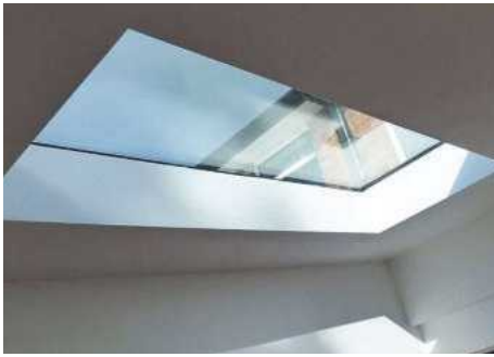
A flat roof light
