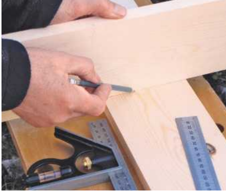
1 Saw timber to length and mark positions of housings on side pieces; mark both together as a pair
