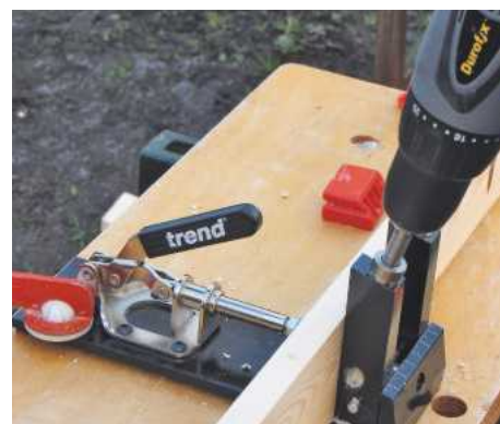
18 Fix stretchers with pocket-hole screws, using a suitable jig to drill the holes. Next, glue and cramp stretchers to the shelves while inserting screws
