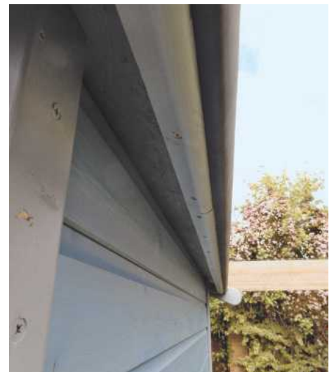
25 Here you can see the under eaves trim holding the rubber membrane in place
