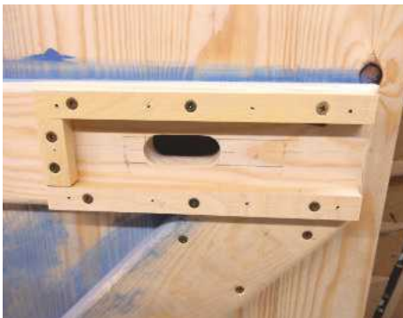
7 Initially, I thought of fitting a metal latch but as these tend to have sharp edges, I opted for a wooden one, and rounded the edges myself
