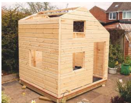
3 The side panels are relatively straightforward: one is 1.5m high and the other, with a window opening, 1.8m high
