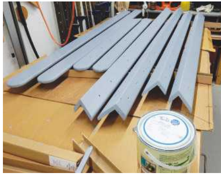
20 All external capping and trims were prepared and, where appropriate, edges rounded over. Two coats of grey paint were then applied – here you can only see the fascia boards and corner trims, but I assure you there was a lot more to it!
