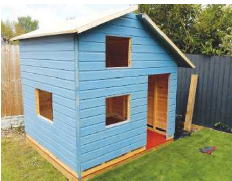
23 Transporting the completed flat-pack proved a little trickier than originally planned, and due to the size of panels, instead of a van I ended up with a flat-bed vehicle
