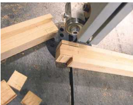
17 Use a saw to remove most of the waste
