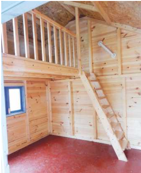
26 Fitting out the inside didn't take long as everything was pre-finished and all holes pre-drilled
