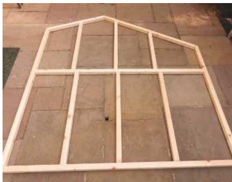
1 The frames for the front and back are similar but not identical as only the front has a door and windows
