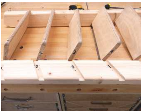
15 After rounding over all side rails edges and front and rear edges of the treads, the stairs could be dry assembled
