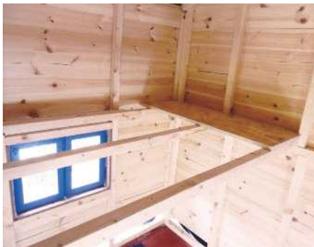
13 Internal fit-out started with the mezzanine floor. Three 'joists' support a 3/4" OSB floor, which is made up from three pieces
