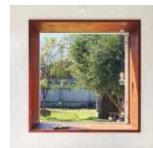
A timber window reveal
