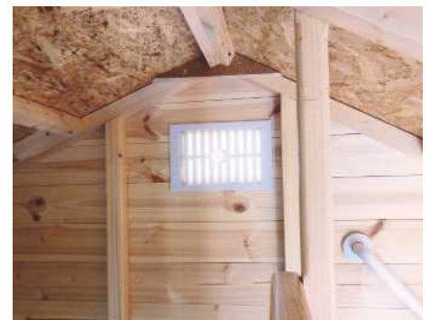
30 A further addition was an air vent with insect screen located in the rear wall – it gets quite hot inside the playhouse when the sun shines
