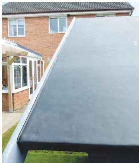
24 The roof is covered with Firestone EPDM rubber membrane, which is largely intended for flat roofing but can also be used on sloping roofs
