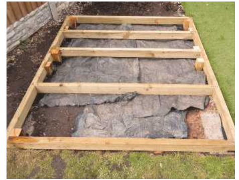
21 On site at my daughter's house, the first task was to install the base frame
