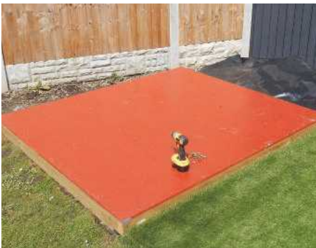
22 Next, the floor panels were screwed down. These had previously been painted on both sides with two coats of floor paint, effectively sealing the surface
