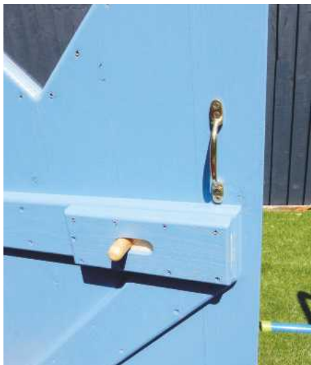
29 ... and a solid brass handle added inside the door to assist closing
