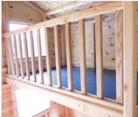
27 The mezzanine floor was covered with a piece of industrial vinyl flooring leftover from a camper van build. Here you can clearly see all rounded-over edges on the rails
