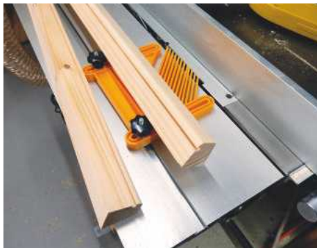
12 Drip caps – for placing over the door and opening window – were made from some 2x2in scant. Using the table saw, I ripped a slope on the top edge and created a drip rebate on the underside
