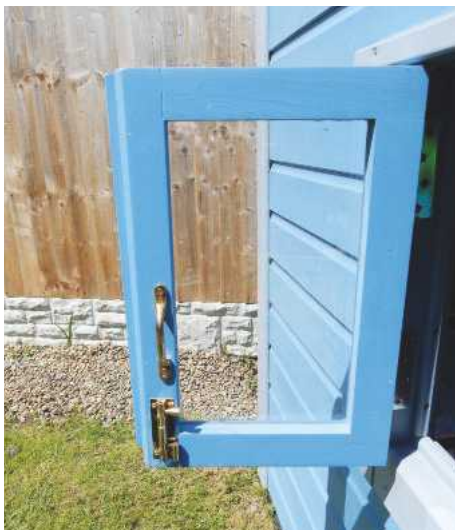
28 A solid brass handle and lock were added to the inside of the opening window...
