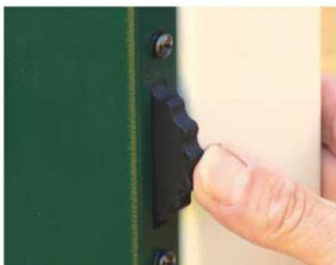
Both upper and lower steel doors are locked with circular knobs, which operate well
