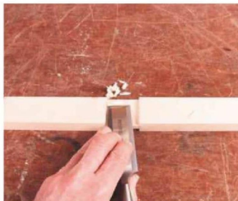
13 Clean up the base of the joint with a wide-bladed chisel. If you don't have a router, use this to pare away all the waste
