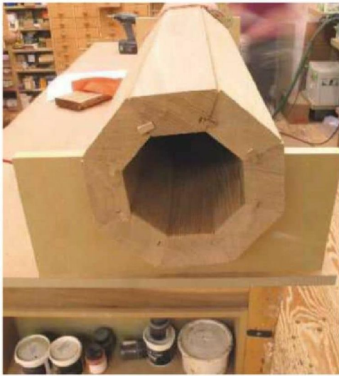
1 The porch columns are made from kiln-dried European oak. I start by drawing out a section according to the dimensions, then machine it. The angle on each is 22.5°
