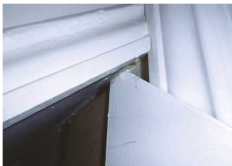
24 Detail trimmed to allow door to open
