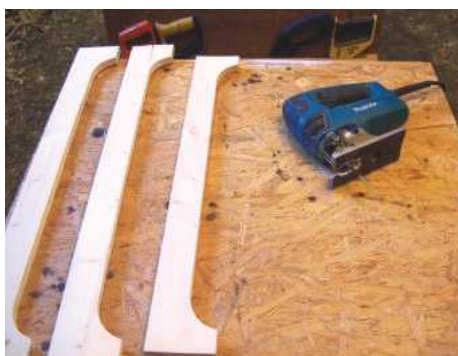
4 The support rails are cut and fluted
