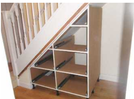
16 The frame in situ with the plinth leg
