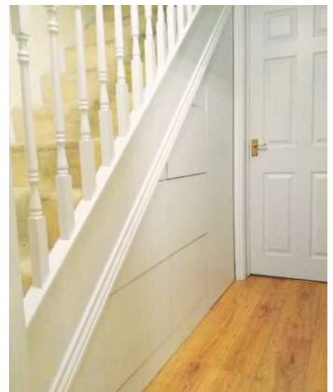
25 The completed understairs storage solution
