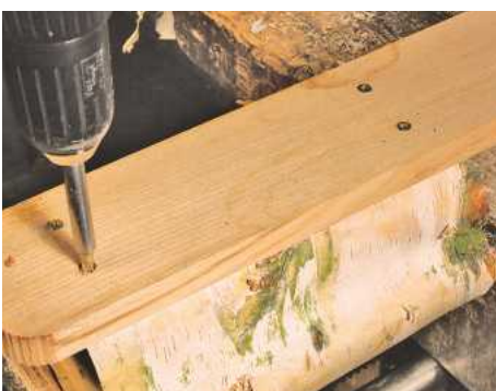
12 Cut the backplate to size and screw it securely to the back of the box
