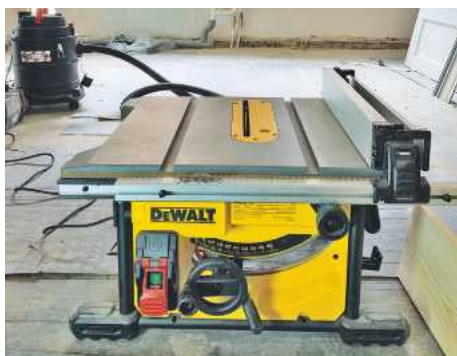
The table saw set up on site
