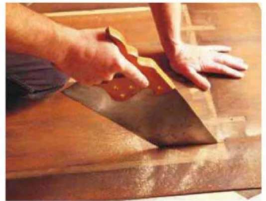
10 Ripping the oak table top into its component boards
