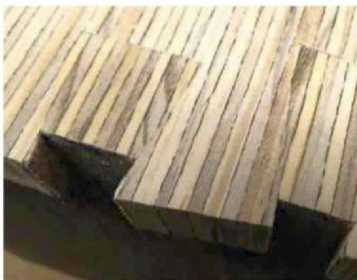
6 So much for continuation of grain – the joint is lost!
