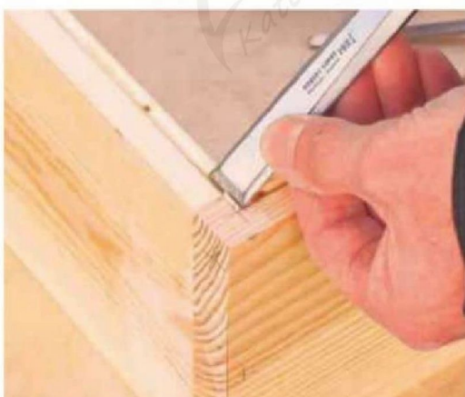
8 The position where the beading intersects at each corner will need tidying up. Do this with a sharp chisel
