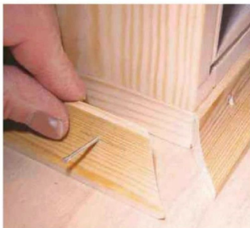
23 Fit the front piece of coving first, pre-drilling before pinning to the blocks
