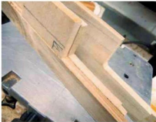
17 Note the use of straightedge guides to form a neat finish on the window frames
