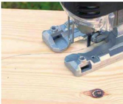
2 Carefully cut out the curves with a jigsaw, ensuring to keep just on the waste side of the pencil lines
