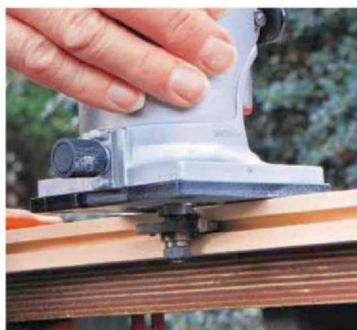
12 Rout a groove along the inner edges of the door stiles and rails. The MDF panel should be a sliding fit
