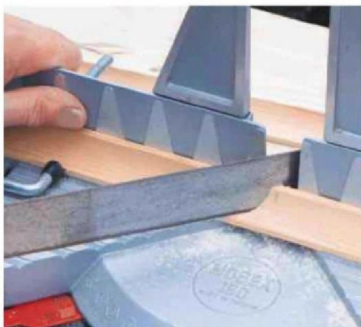
22 Saw the coving to length with a mitre saw, and trim with a block plane if slightly over length
