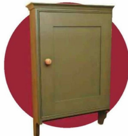
24 Mark and drill fixing holes in wall and lift cabinet into position. Fill pin holes, then sand and paint
