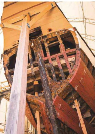
21 Framework at the stern of the ship
