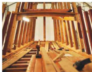
17 Work on the interior and cabin
