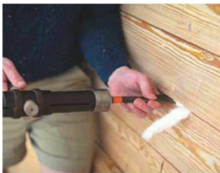
28 Caulking is essential to ensure everything is water-tight
