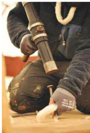
26 Using the caulking hammer
