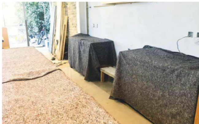
All done for the week on site – everything covered in blankets to protect it from ongoing renovation work in the house
