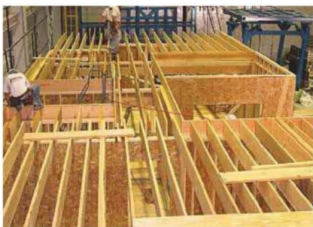
The installation of floor joists
