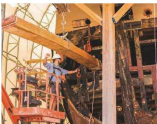
22 Heavy timber being passed through the exposed stern of the ship
