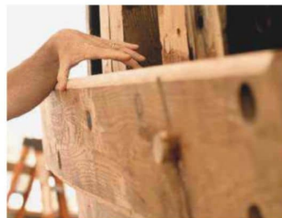
7 Wooden trenails, also called 'treenails' or 'trunnels'
