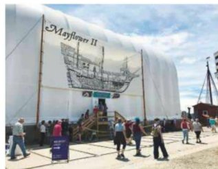
5 Temporary shelter nicknamed 'the mailbox' where restoration work took place
