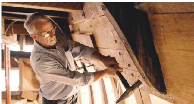
14 Securing a knee below deck
