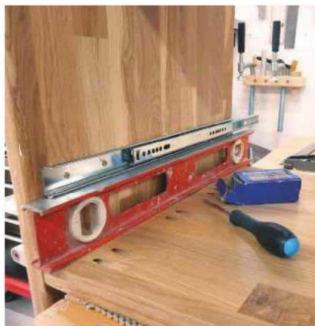
13 Installing the drawer slides
