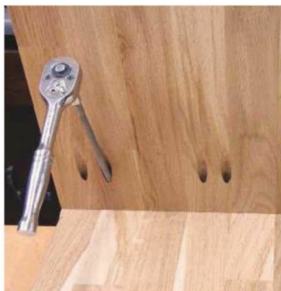
16 Checking screws are tight
