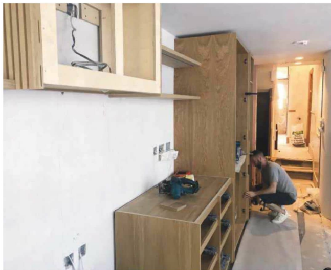
Barry, the experienced fitter, screws a cabinet divider in place
