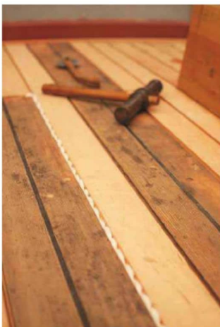
25 Caulking the deck
