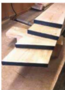
Timber with DPM fitted
