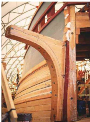
9 Cathead replaced this horizontal beam used for raising the anchor
