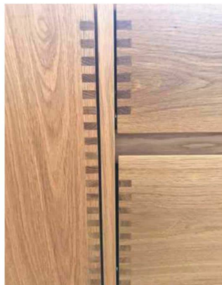
All of the drawer and cabinet fronts feature these eye-catching finger joints. Even the backs of the drawers, too!
