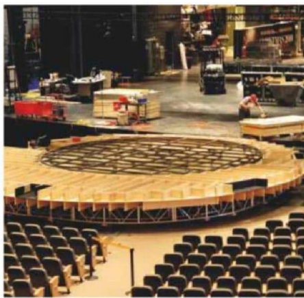
A wooden revolving stage with turntable
