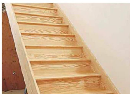
Housed stringer stairs
