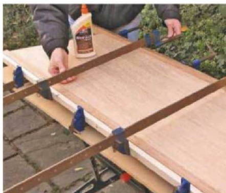
11 Prepare lipping slightly oversize from solid oak and glue to front edge of the MDF window board
