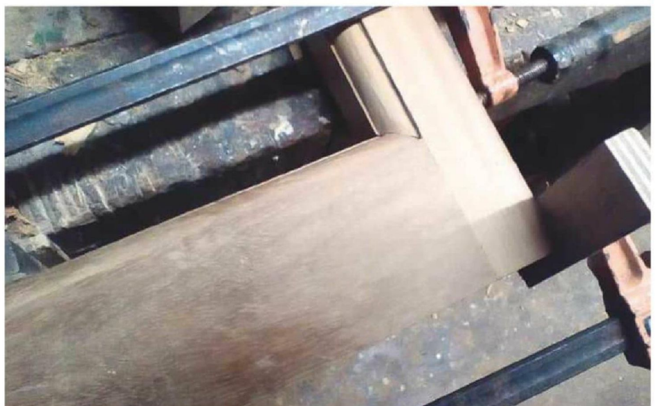
6 Replacement window, glued and clamped up
