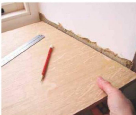
10 Check MDF fits into the opening and adjust if necessary. True up the front edge with a bench plane
