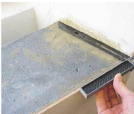
4 A template is necessary for making a window board that fits snugly. Use a sliding bevel to transfer the angle
