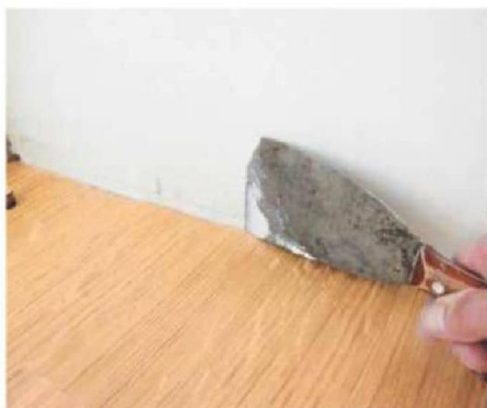
22 Fill gaps in masonry next to window board and sand down. A second application may be necessary
