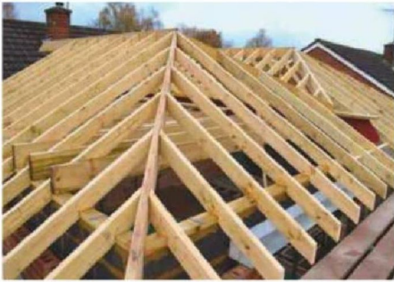
Hip joints on a roof
