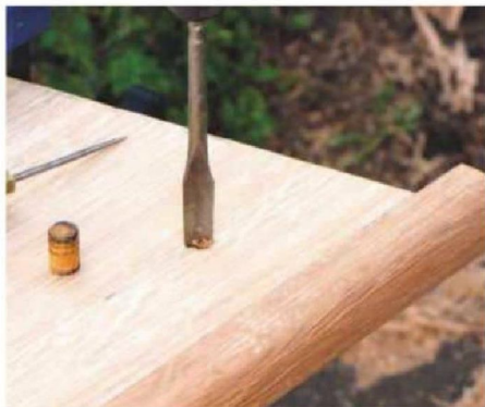
16 Mark screw positions and counterbore to accommodate matching oak plugs. Drill for 5mm screws
