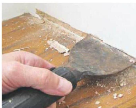
2 Chop away plaster around timber with a cold chisel. Drill through plugs, unscrew and remove the existing window seat
