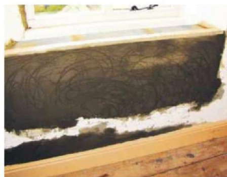
3 Wall height has been increased with the new blockwork. After rendering and plastering it can then be painted
