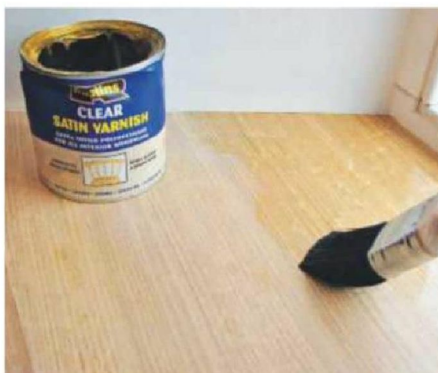
23 Lightly sand again and brush on a couple of coats of satin polyurethane varnish, thinning the first one
