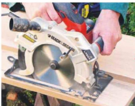
7 Cut MDF board to correct depth with a circular saw, running the tool against a straightedge for accuracy
