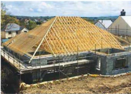
Hipped roof designed and built by Melingoed LTD
