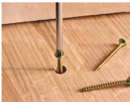
19 Mark and drill blockwork, then insert wall plugs. Fix window board in place with 5mm screws
