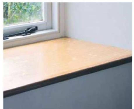
24 The deeper lipping actually makes the completed window board look more substantial
