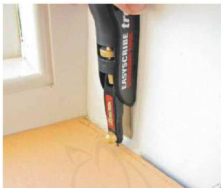
5 If walls are uneven use a scribing tool to mark the card accurately. Tape two lengths together if you find it is short
