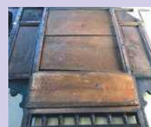
The back of the mirror showing damage
