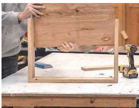
22 Sliding one of the drawer bottoms into place
