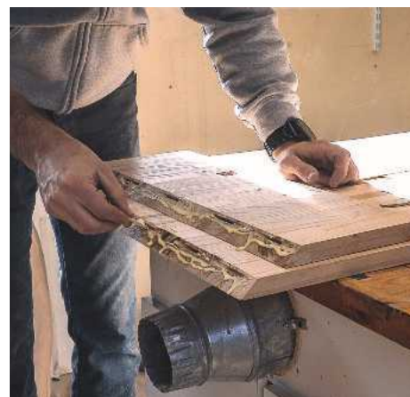
13 Applying a generous application of glue to the pockets, biscuits and entire corner
