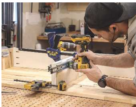
19 Mounting the drawer slides to the desk
