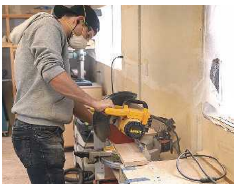
3 Using painter's tape to mark the different lengths worked really well
