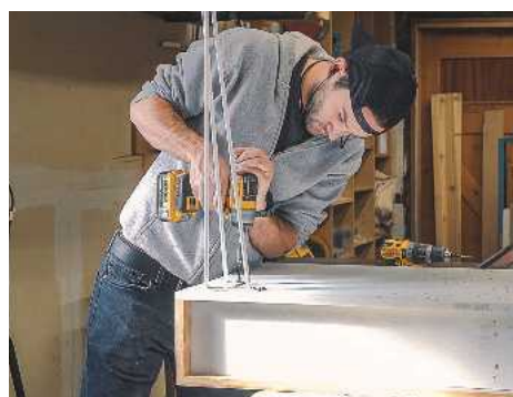
28 Installing the hairpin legs using some No.10 20mm pan head screws
