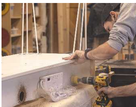
29 Mounting the power strip to the backside of the desk
