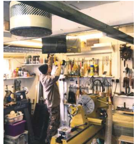
Fixing some of the materials in place
