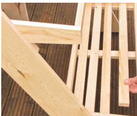
26 Saw remaining slats to length so they're a loose fit in shelf trays; sand and remove the arrises
