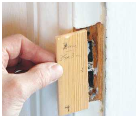
7 For a neat job, cut softwood blanks slightly oversize; glue in place and trim flush with a shoulder plane
