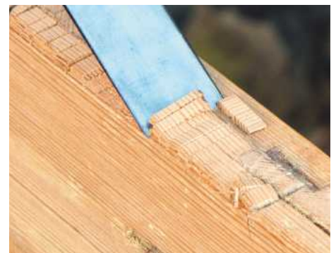
5 Carefully cut a new recess with a chisel; check the lock fits and glue a softwood blank to fill the old cavity
