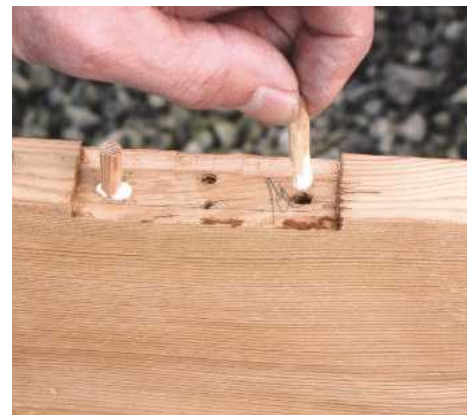
6 Not all screw holes will line up with the new hinge position so carve small plugs, glue and tap into the old holes
