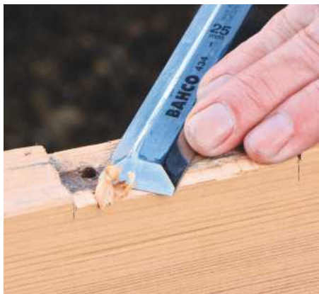
5 Pare down to the gauge line and check the recess is flat with a small square; trim ends and check the hinge fits
