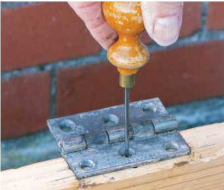
7 Mark centres of new holes with a bradawl; drill and screw flap to door edge; repeat for second hinge
