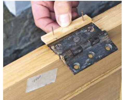
9 Cut and glue wood strips to cover the edges of the old hinge recess; remove pins when dry and trim flush
