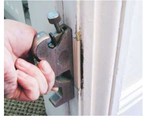
15 Fill old hinge recesses in the same way, pinning softwood until the glue is dry; trim flush with a shoulder plane
