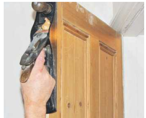
12 You'll need to plane the door edge if it binds when closing; remove door to plane if the lower edge binds
