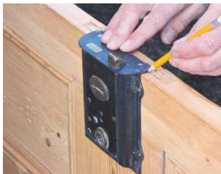
4 Place the rim lock on the reverse side of the door and draw around the plate, making sure spindle holes line up
