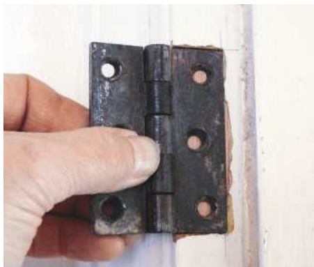
11 Clean up recesses with a chisel and check hinges fit snugly; chipped paintwork will be sanded later
