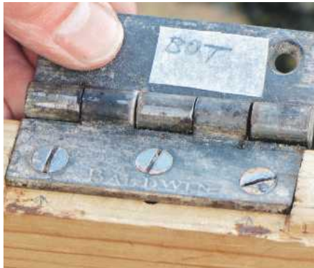
8 It's wise to label hinges with masking tape so they don't get mixed up – screw holes don't always match
