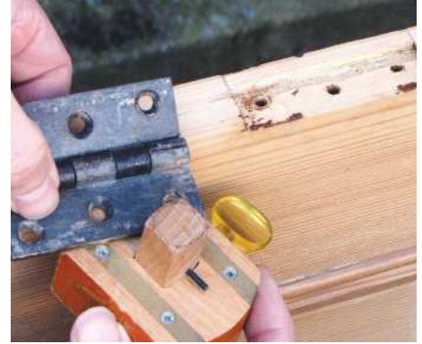
3 When reversing hinges, set the marking gauge to the thickness of the hinge flap, then mark the depth on the edge of the door
