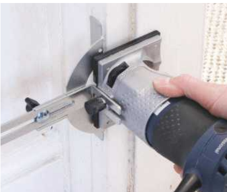
10 Mark new hinge recesses on the jamb – chop out with a chisel or carefully rout away most of the waste
