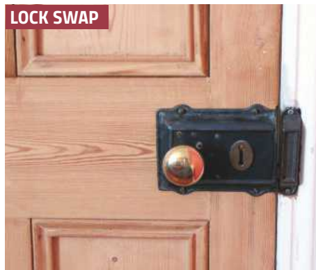
1 A rim lock is easier to swap than a mortise lock, though its box keep still leaves a cavity
