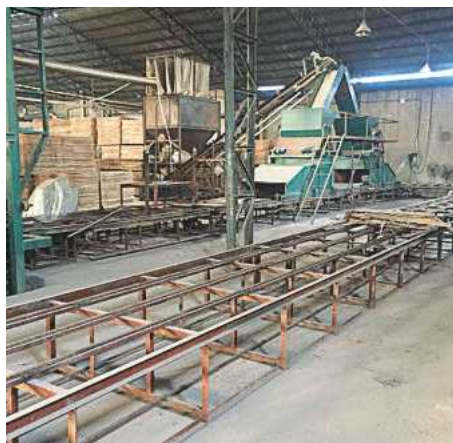
Medium density fibreboard production line
