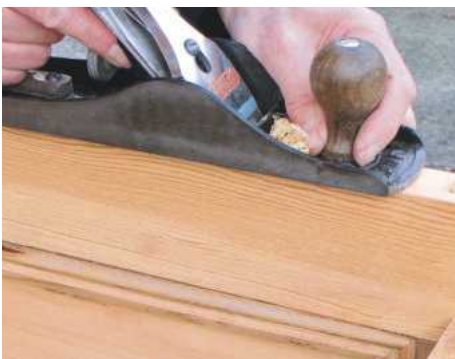
3 Remove the door and check for fit between jambs. Shoot if tight, but be economical when planing
