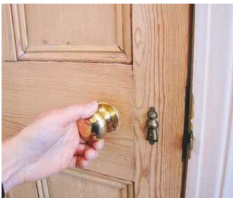
16 Check the latch engages properly; fill holes and small splits and tint new wood that will stay unpainted
