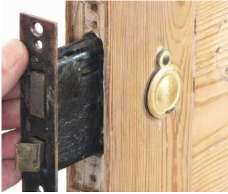
13 Remove mortise lock from the door; to reverse its operation, unscrew the metal case and swap the latch over
