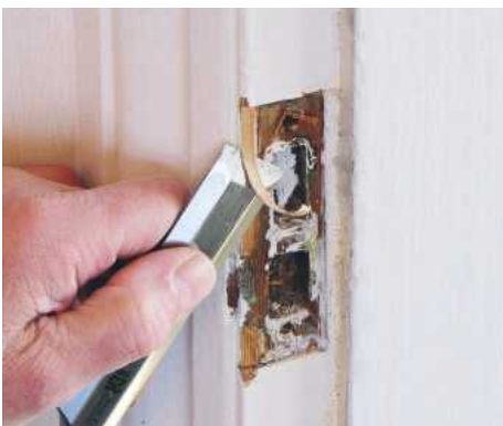
6 Clean off paint from old hinge and lock recesses with a chisel; aim to get wood as flat as possible
