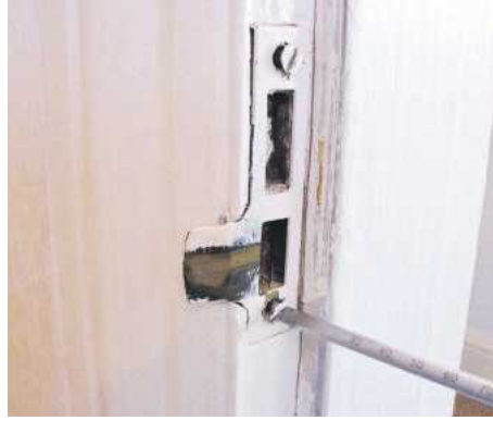
14 Unscrew the striking plate and chop the mortise on the opposite jamb; cut a softwood block to fill the cavity, then glue
