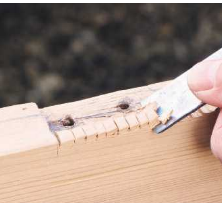
4 Make a series of vertical cuts with a chisel into the wood adjoining the recess, then remove the waste carefully
