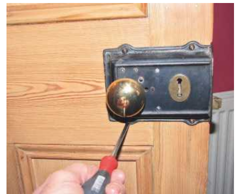
2 Brass door knobs are usually secured with fiddly grub screws; once removed, unscrew the rim lock
