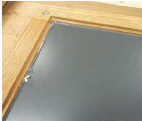
10 Push points and silicone to hold glass in place
