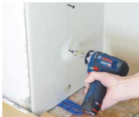
18 Continue cutting and fitting plasterboard around the inside of the alcove. Measure and mark positions of studwork to provide a solid fixing
