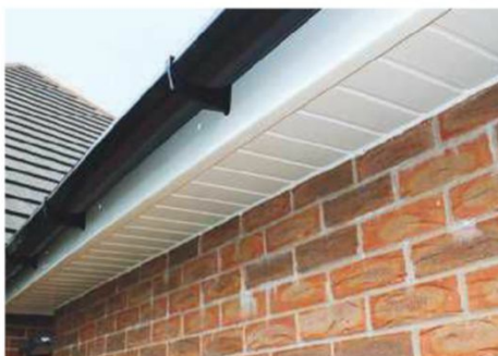
Soffit boards are located on the lower, outer end face
