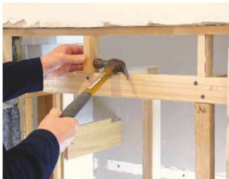
13 Wedge short pieces above the framework to give extra support for the plasterboard. Secure with L brackets if screws are tricky to drive in
