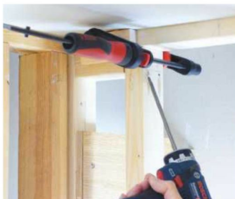
17 If necessary, it's easy enough to add extra studs by using pocket hole screws. These will give support for the floating shelf brackets
