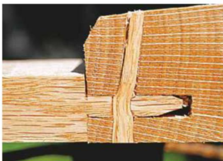
Drawboring demystified: this ancient mortise & tenon joinery technique requires no glue or clamps Photograph courtesy of Popular Woodworking
