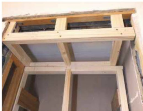
14 It may seem over-engineered, but the framework needs to be substantial enough to support the weight of the loaded shelves in the alcove
