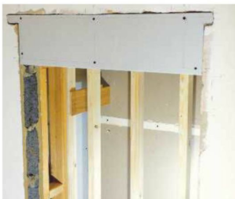
16 Fix the plasterboard to the framework with drywall screws. Screw heads should be just below the surface to avoid fouling the trowel
