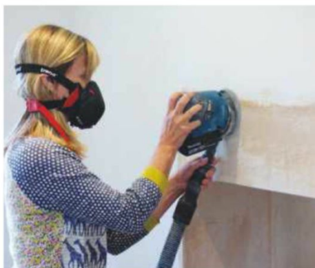
19 Once the alcove is boarded out it can be skimmed with plaster. Leave to dry for a few days before sanding edges flush with the existing wall
