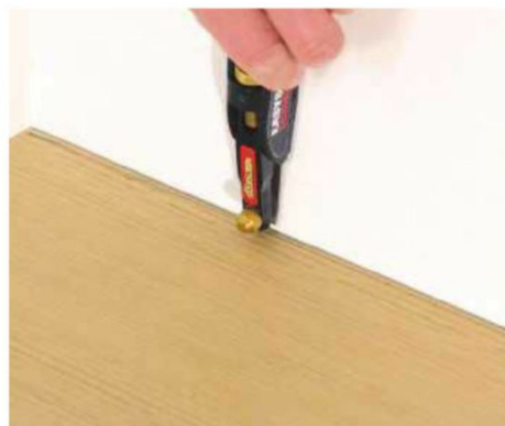
24 Slide the shelf into the opening, trimming the sides if too tight. Use a scribing tool to mark the rear edge of the board
