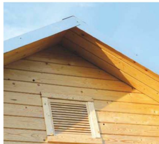
Fragment of just-installed wooden roof eaves with ventilation grille
