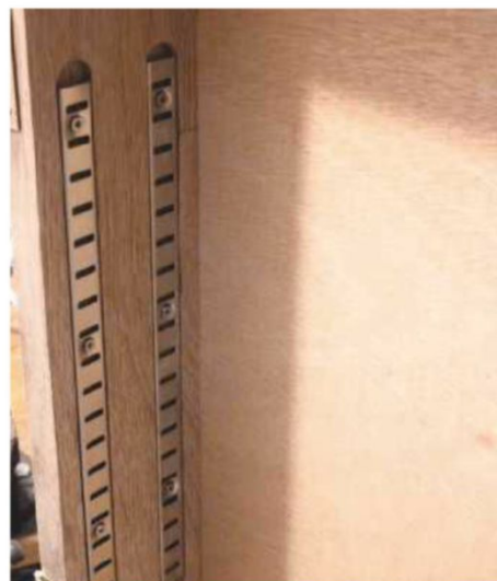
4 Shelf support strips in routed slots
