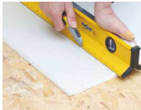
15 Mark and cut the plasterboard to fit around the inside of the alcove. Use a sturdy straightedge when cutting with a craft knife
