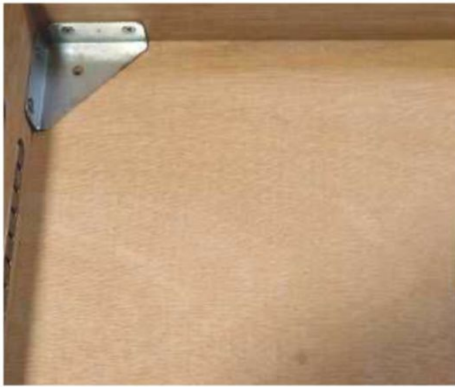
6 Triangular support brackets screwed into carcass
