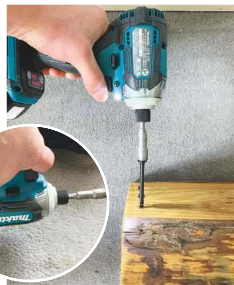
Inserting a Tekscrew into oak
