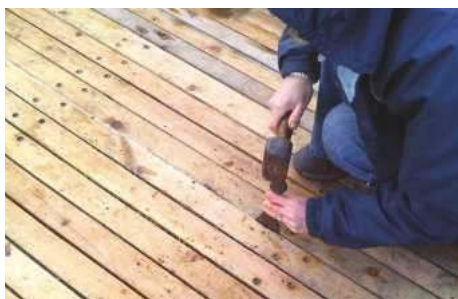
Caulking a wooden deck
