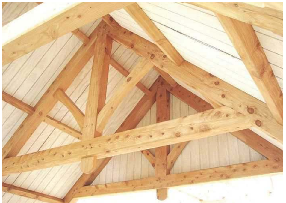
Collar-tie roof truss joint
