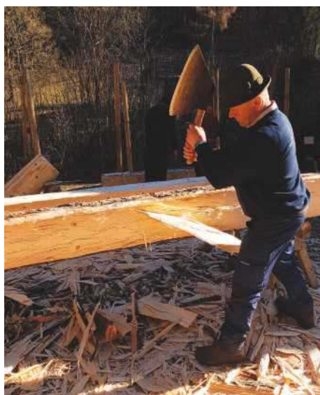
The finishing broad axe in action
