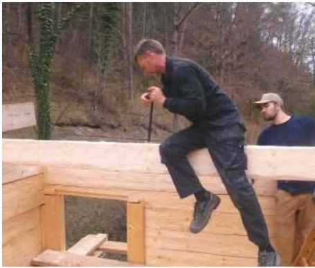
Drilling peg holes for locating the next beam
