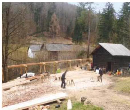
Hewn logs ready for assembly
