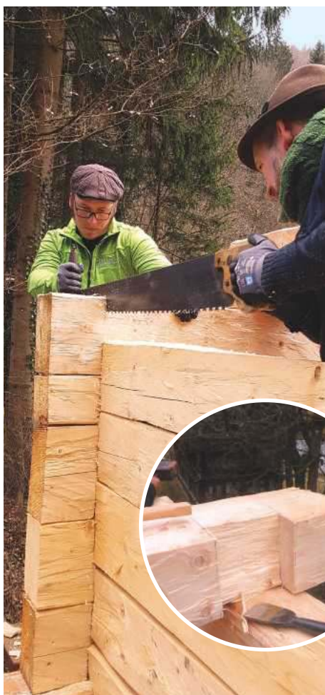
Cutting a halving joint
