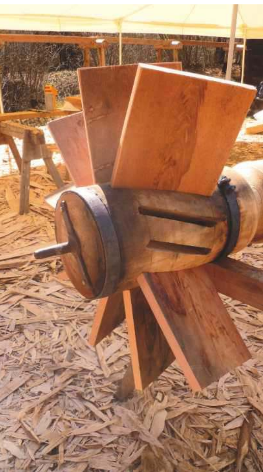
Fitting paddles to the mill shaft
