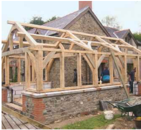
Timber frame extension
