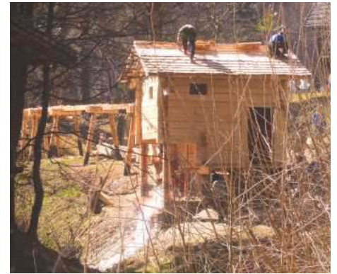
Fitting shingles to the roof
