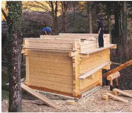
Building up the walls
