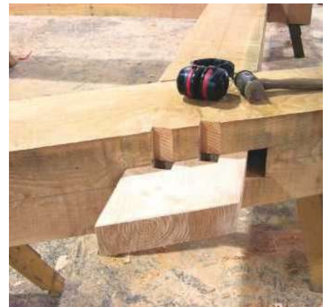
16 A-Frame wedged and keyed with traditional joinery
