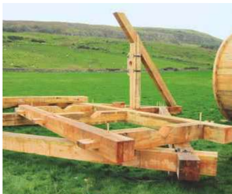
11 Chassis and ladder frame assembled on site
