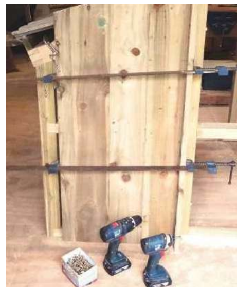
2 6 by 1 (150 × 25) sawn tanalised softwood is rough stuff. It will expand and contract with the weather, but to give it its best start, I cramped before screwing. Just visible in this photo is a near-mistake. I have the side frame screwed to the back frame from the outside. When that last plank is fixed, I wouldn't be able to dismantle for transport. Duh! Now it is screwed from the inside
