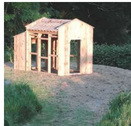
5 Initial assembly. I could have clad it indoors, but I wanted to be sure that I could move it; and I wanted to be able to stand back from it to see it properly. Now I think the doorway might receive a drip moulding like an eyebrow. That gable end needs a little something
