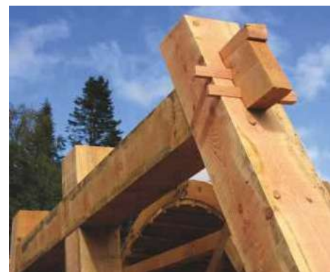
17 Wedged and keyed A-frame
