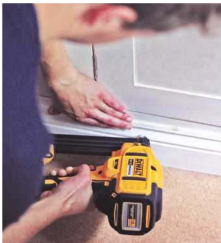
Using the finish nailer to fix a wardrobe kicker plinth in place
