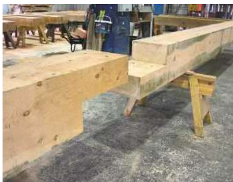
10 The spine beam is scarfed together
