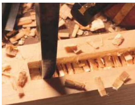
13 The chisel defines the mortise width
