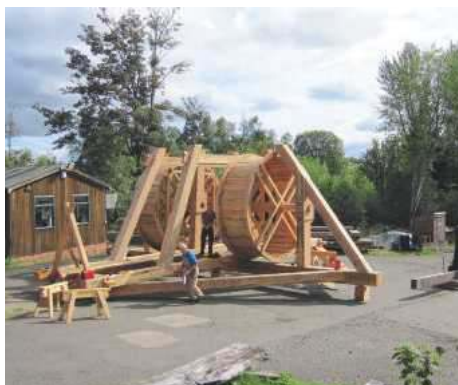
21 The outer axle posts also have supporting diagonal struts to give cross rigidity to the structure
