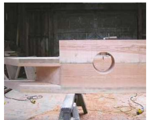
20 Axle block in construction
