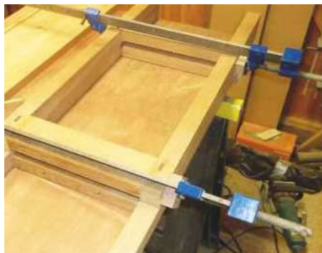
8 The front legs are clamped to the rear to ensure alignment
