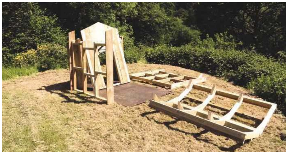
4 More components. I was reluctant to dismantle the roof. I had a long discussion with myself about the sense of lifting this into position, damaging my back and being unable to move for six weeks, then like an improbable weight lifter, I rotated it, lifted it above my head and walked it over three standing sides. Not difficult at all as it happened
