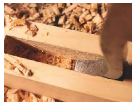
14 A lock mortise chisel levels the floor
