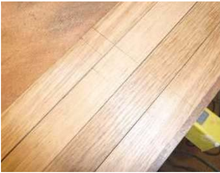
4 Marking out joints
