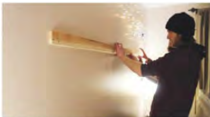
14 Attaching the French cleats to the wall
