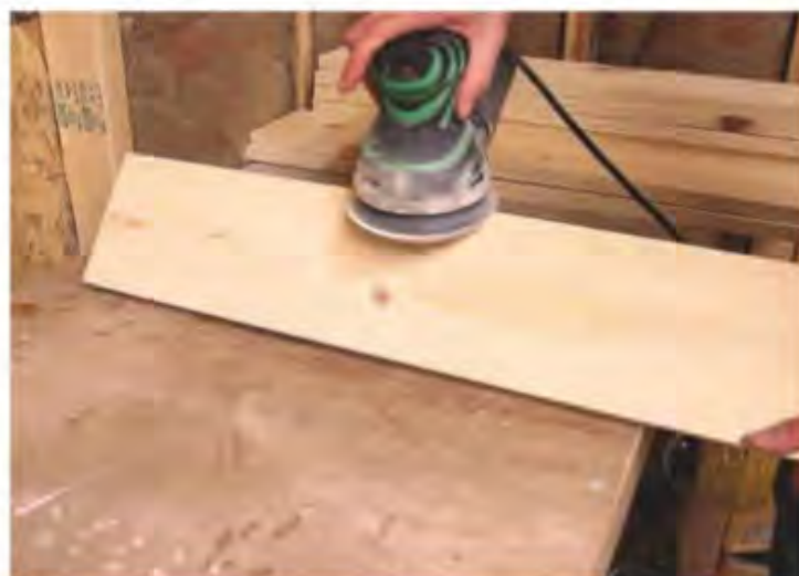
2 Sanding all components up to 220 grit using a random orbit sander
