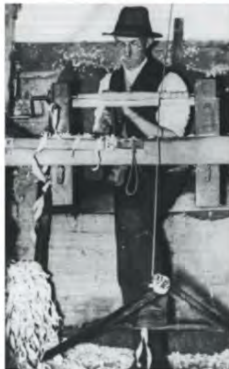
A Bodger at work, making a chair leg on a foot-powered lathe
