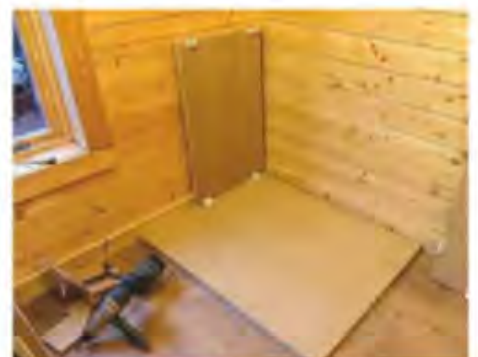
8 Fitting the first side. Again, I used the idea of pushing the work against the (fairly accurately vertical) skirting board when fitting the screws
