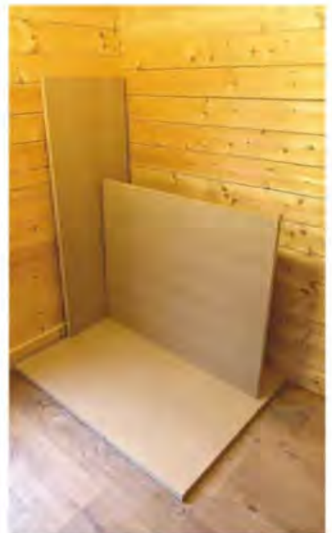
2 And one side. This side piece needs trimming accurately to the height of the infill
