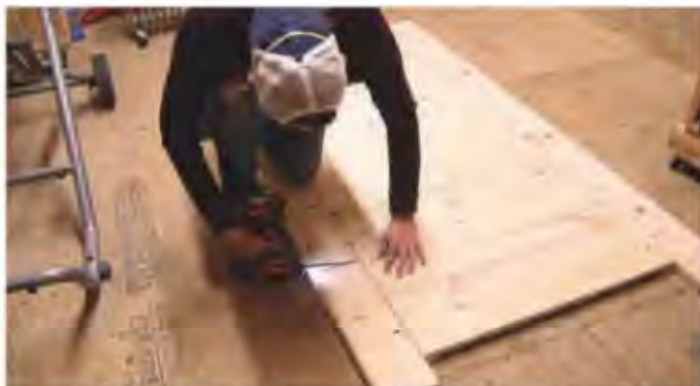
6 Attaching the 38 x 140mm piece to the inside of the headboard using 32mm pocket holes screws
