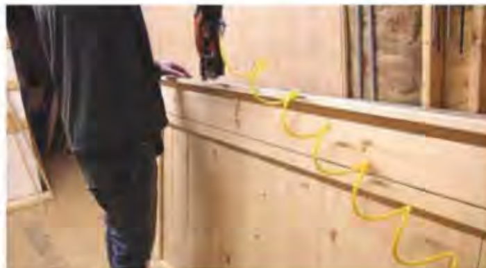
7 Using a finish nailer to attach the top cap
