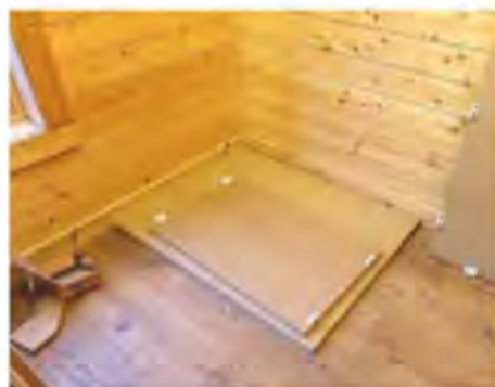
7 Corner blocks on the sides. I used exactly the same process to put four corner blocks on the sides – near, but not too near the corners
