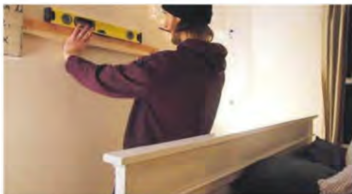
13 Using a level in preparation to hang the headboard
