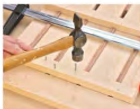
6 Fix battens to the rails using 30mm oval or lost-head nails. Pre-drill ends to prevent splitting
