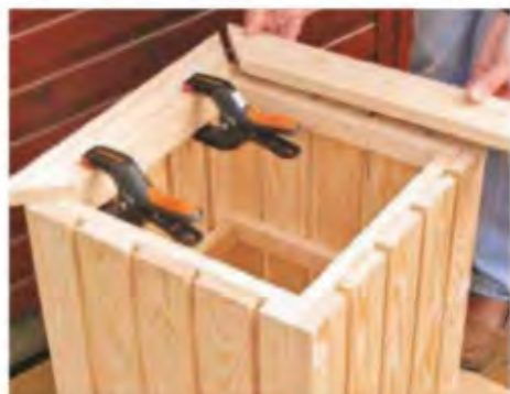
13 Cramp timber in position and cut remaining pieces to size; you could simply cut halving joints if you prefer
