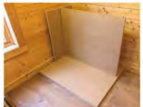
5 The cut side in place. And it fits well – a nice step-less continuous surface. Now it's time to start fitting the corner blocks
