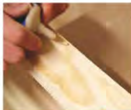
10 Using wood filler to hide the nail holes
