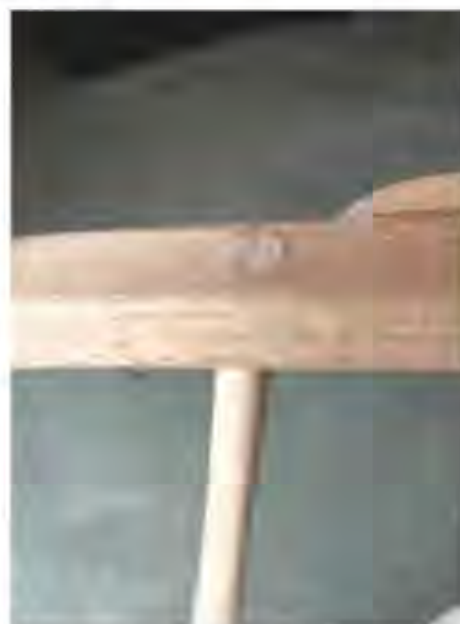
10 Look closely and you will see that the exposed end of this short spindle is slightly larger than below the arm. The wedge has caused it to flare so that it cannot pull back through the hole
