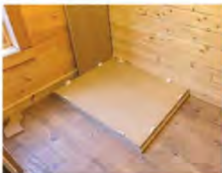
6 Fitting corner blocks. I screwed eight corner blocks on the perimeter of the 'infill' piece. You may see how, at every stage, I have pushed the work against the skirting board in my little log cabin to ensure that I get the edges flush. Now I have to turn over and fit eight more to the other side. I made sure that they were not exactly opposite the blocks on the first side so there was no unfortunate meetings of screws
