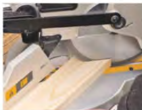
12 The top frame is mitred together at the corners. Cut the first mitre, check timber on the planter and cut the other end
