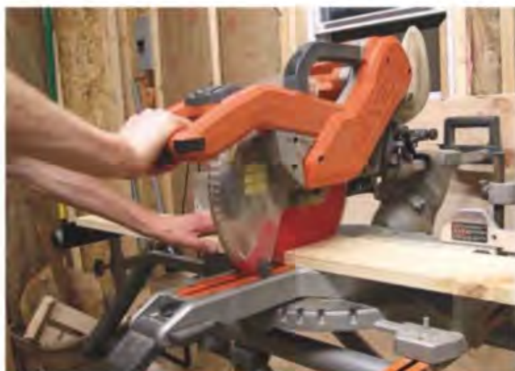
1 Cutting the wood to size using a plunge saw
