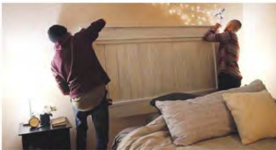
15 Hanging the headboard on the wall
