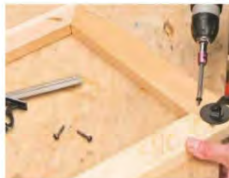
15 Screw the frame together, cramping joints together as you insert the screws. Nail the frame to the top edges of the planter
