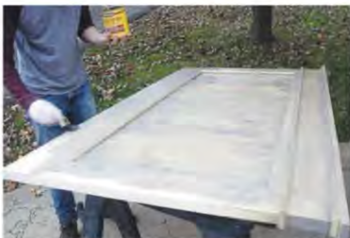
11 Applying the first coat of 'Weathered Oak' stain
