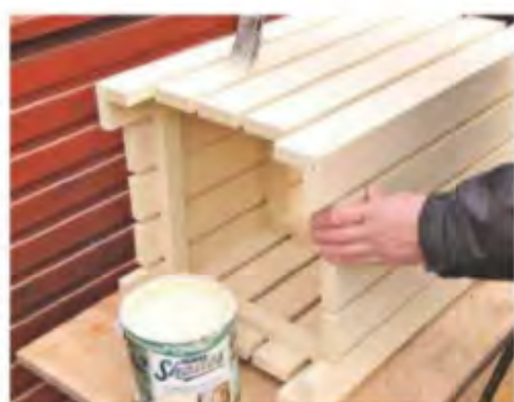
16 Fill nail holes and sand the planter. Brush on a couple of coats of suitable outdoor paint, such as Cuprinol Shades
