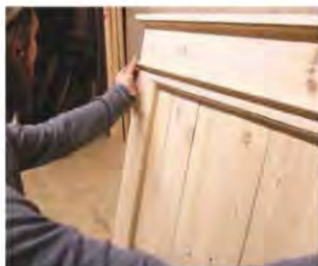
9 Installing a decorative wall trim moulding around the headboard
