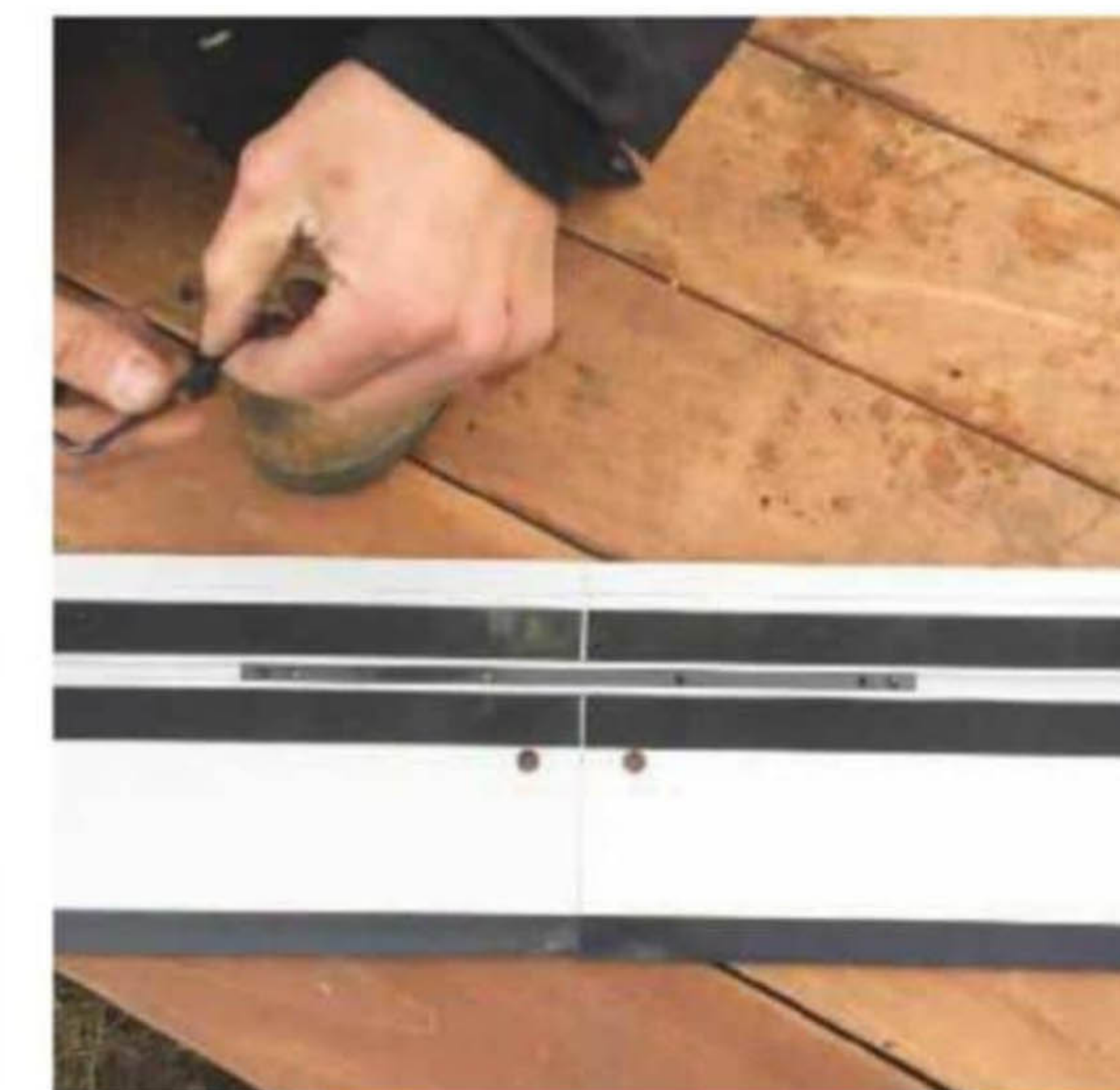
Allen key tightening the connector bar for the rails
