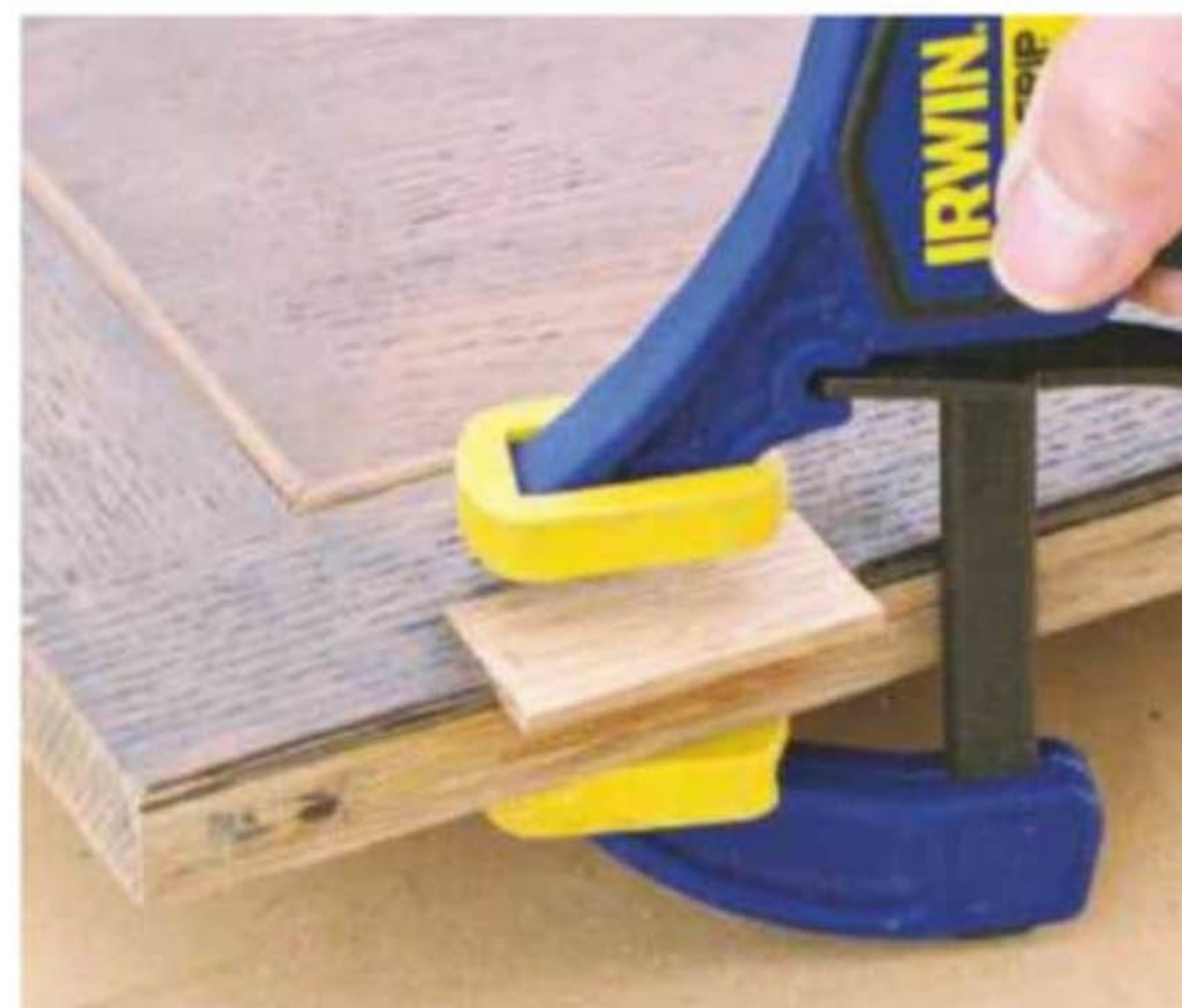
8 Remove door hinges and clean out recesses; cut oak fillets to match and glue in place
