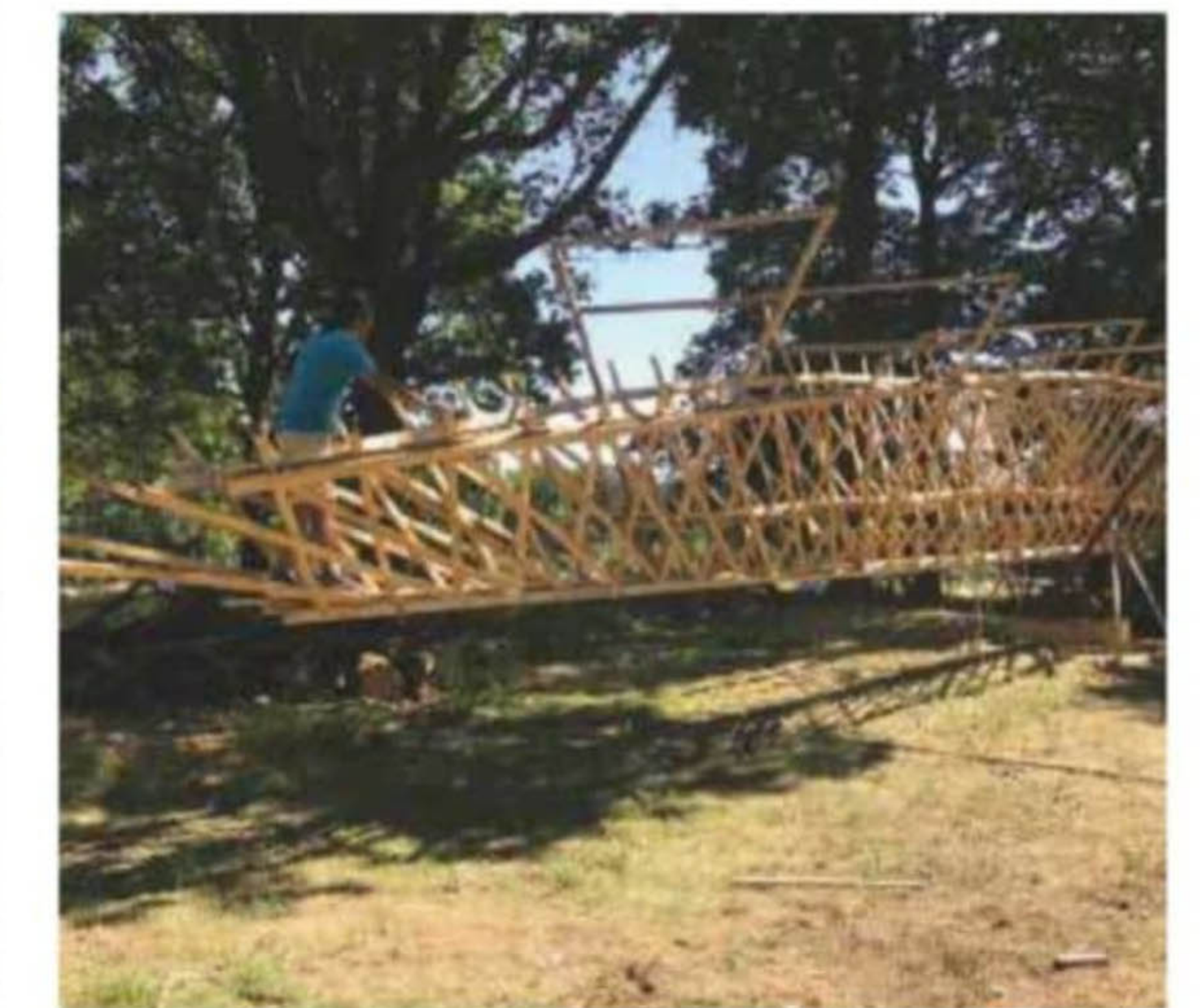
Truss structure being erected by the Cardiff Architectural Students Photograph courtesy of Jim Stephenson
