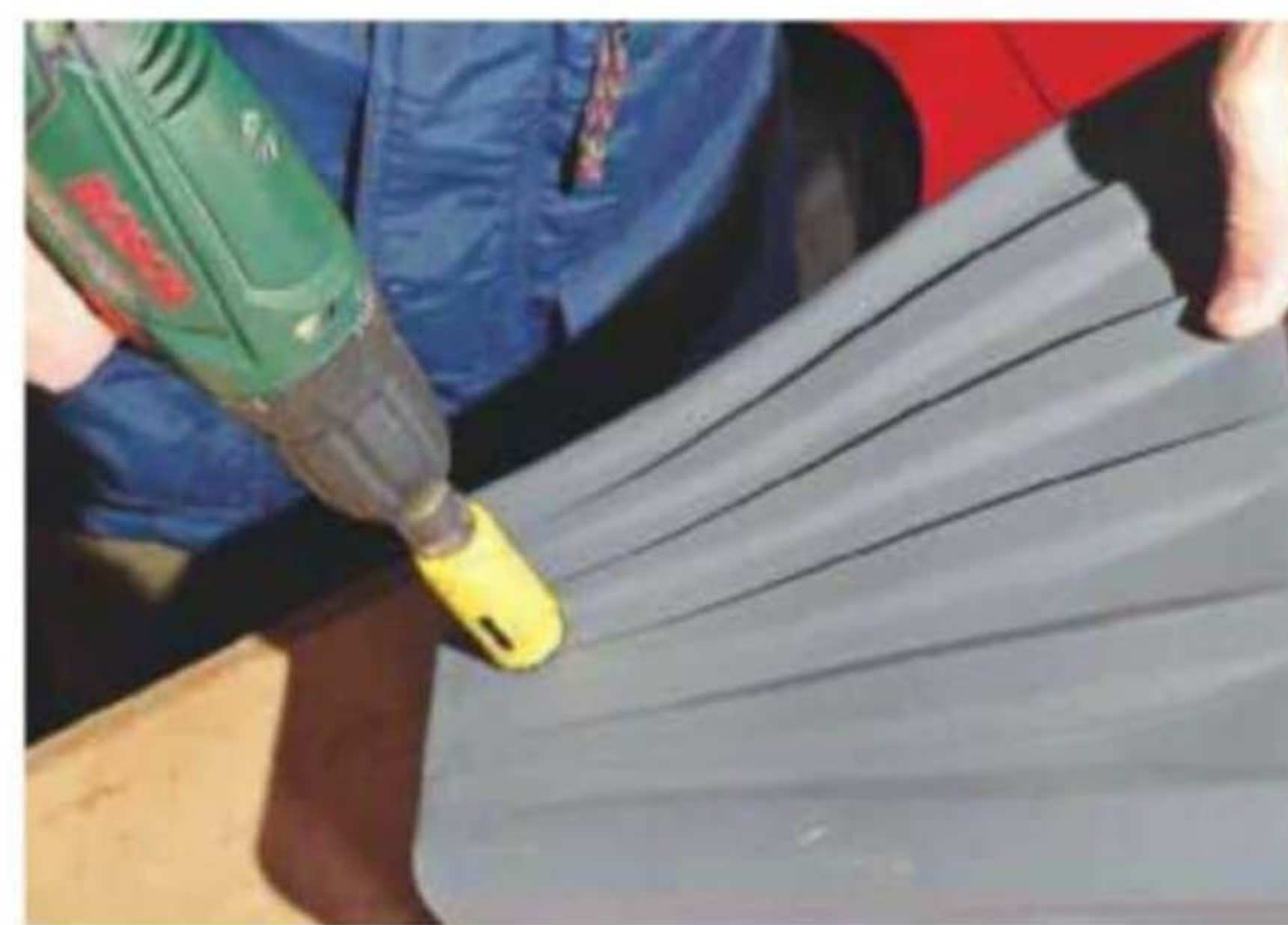
16 Drilling tub for the drainage tap
