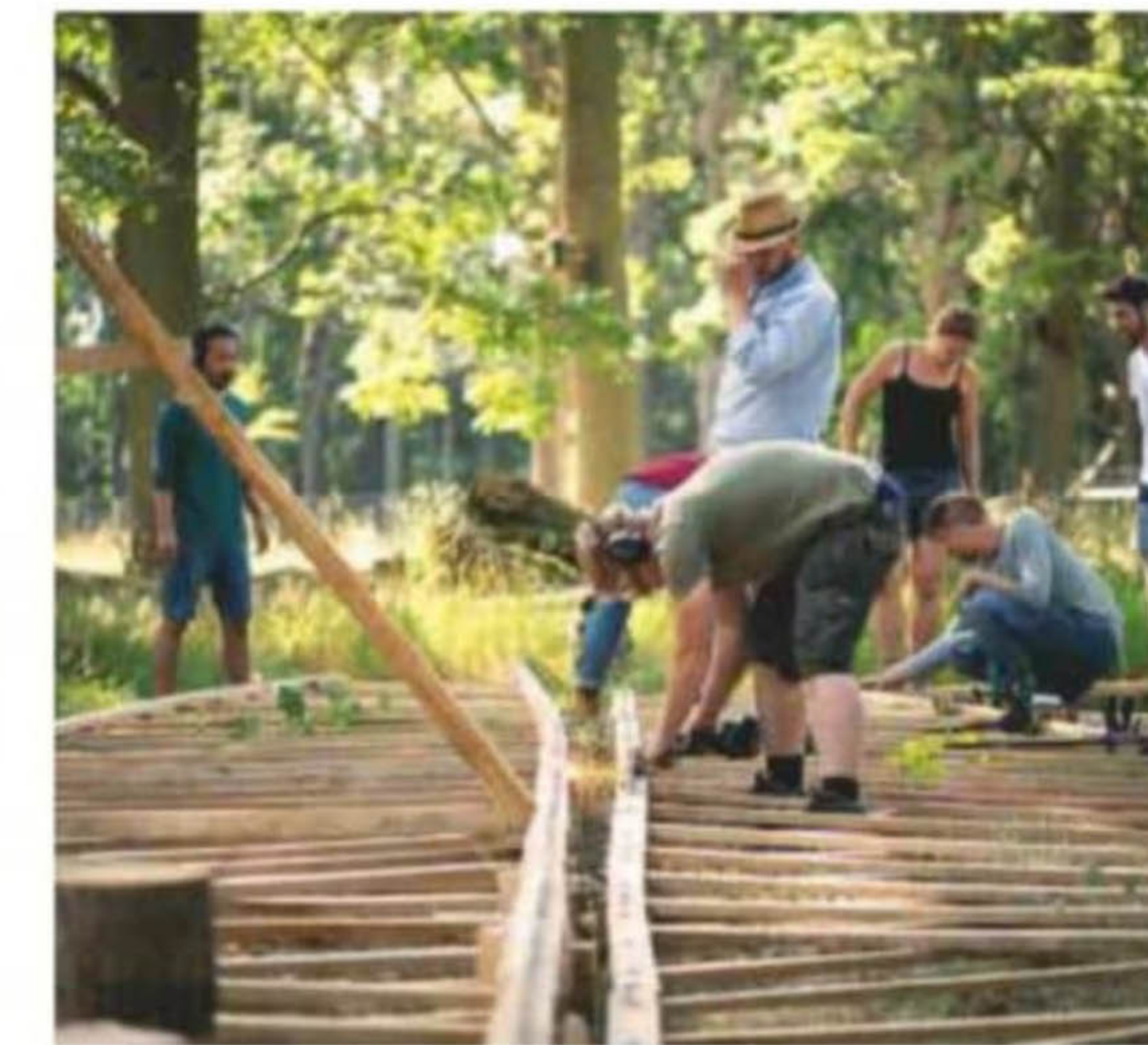
Building various parts for the truss Photograph courtesy of Jim Stephenson
