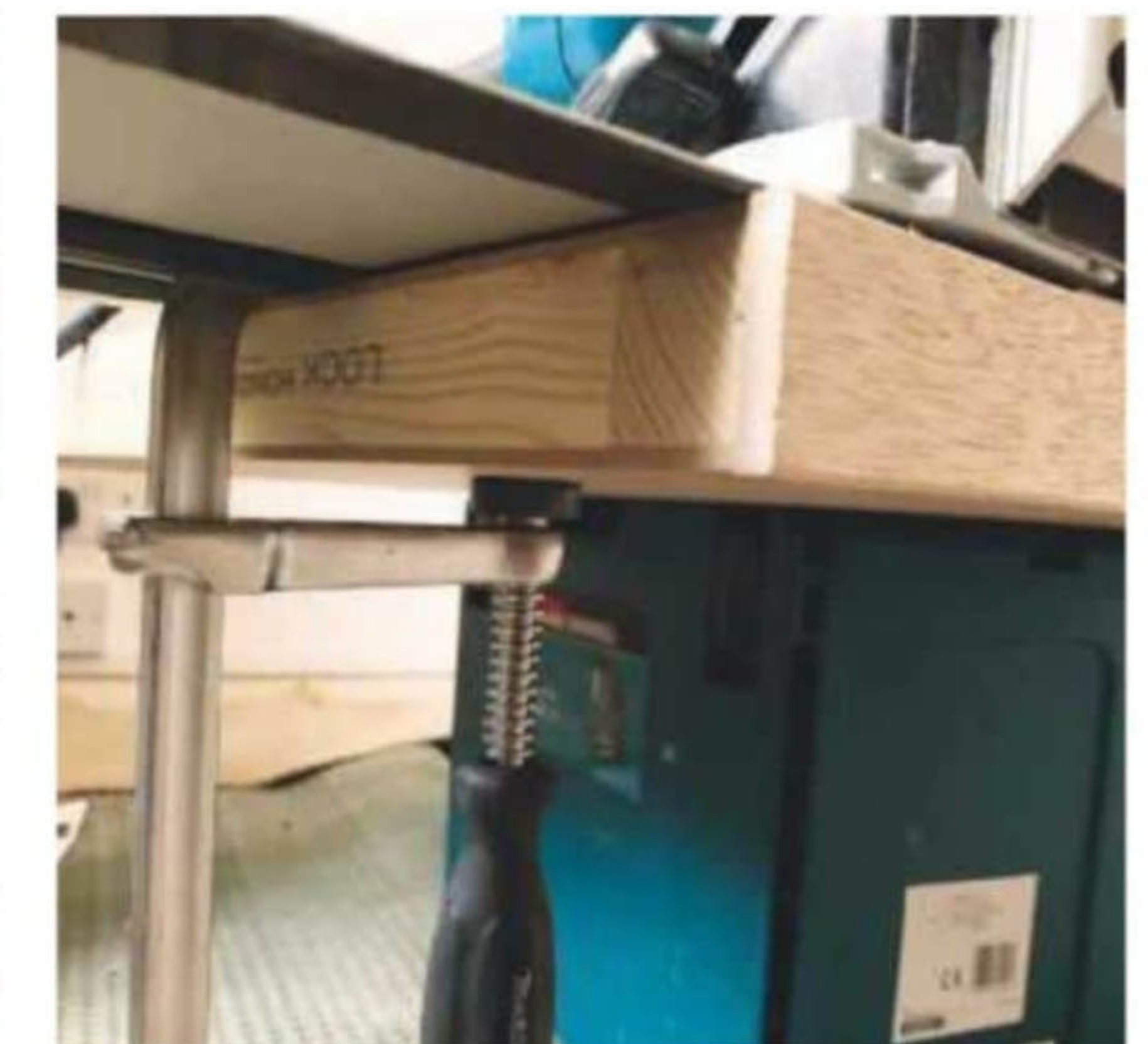
Clamps tightened in position, ready for door to be cut
