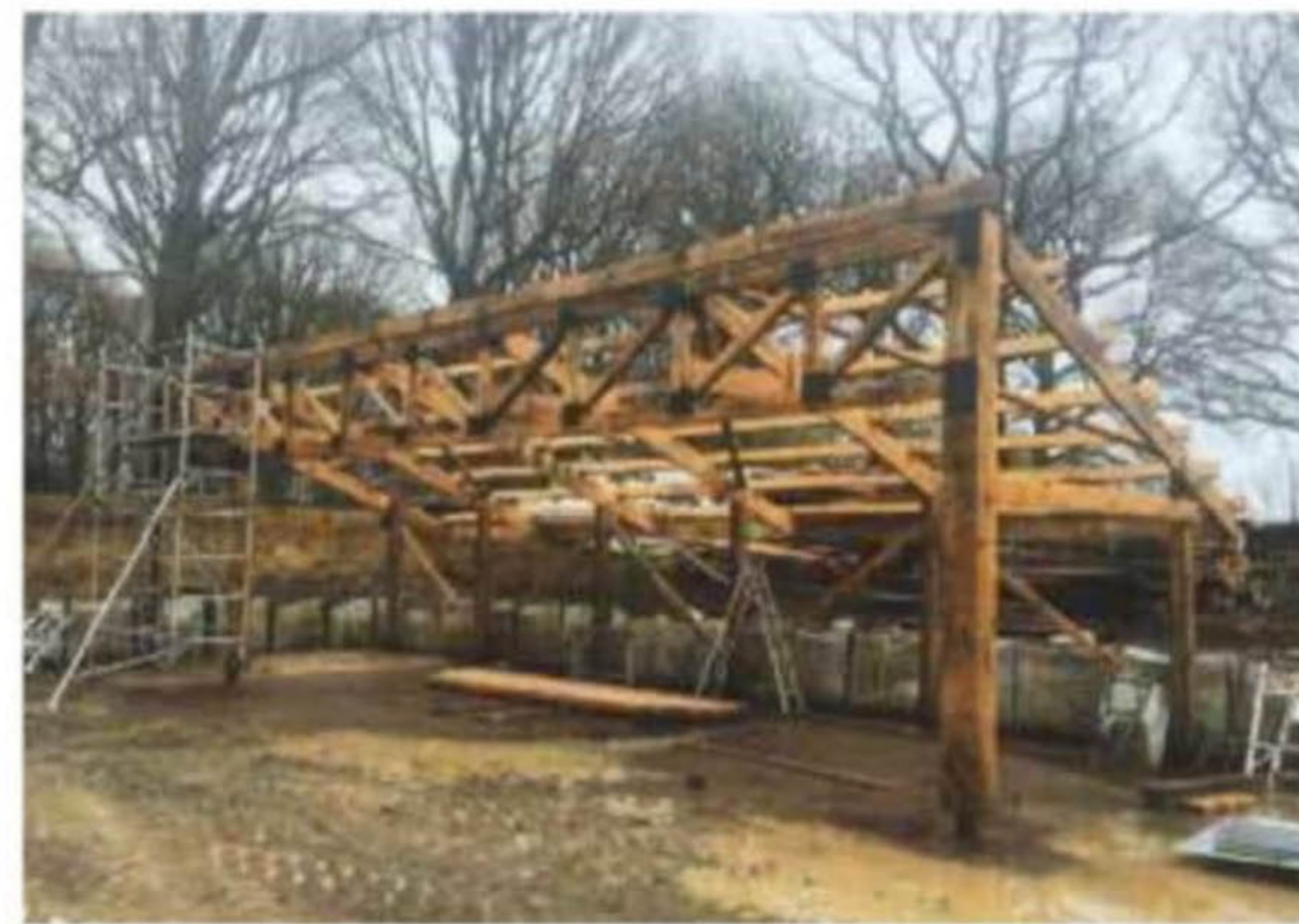
Erecting the sawmill and wood yard
