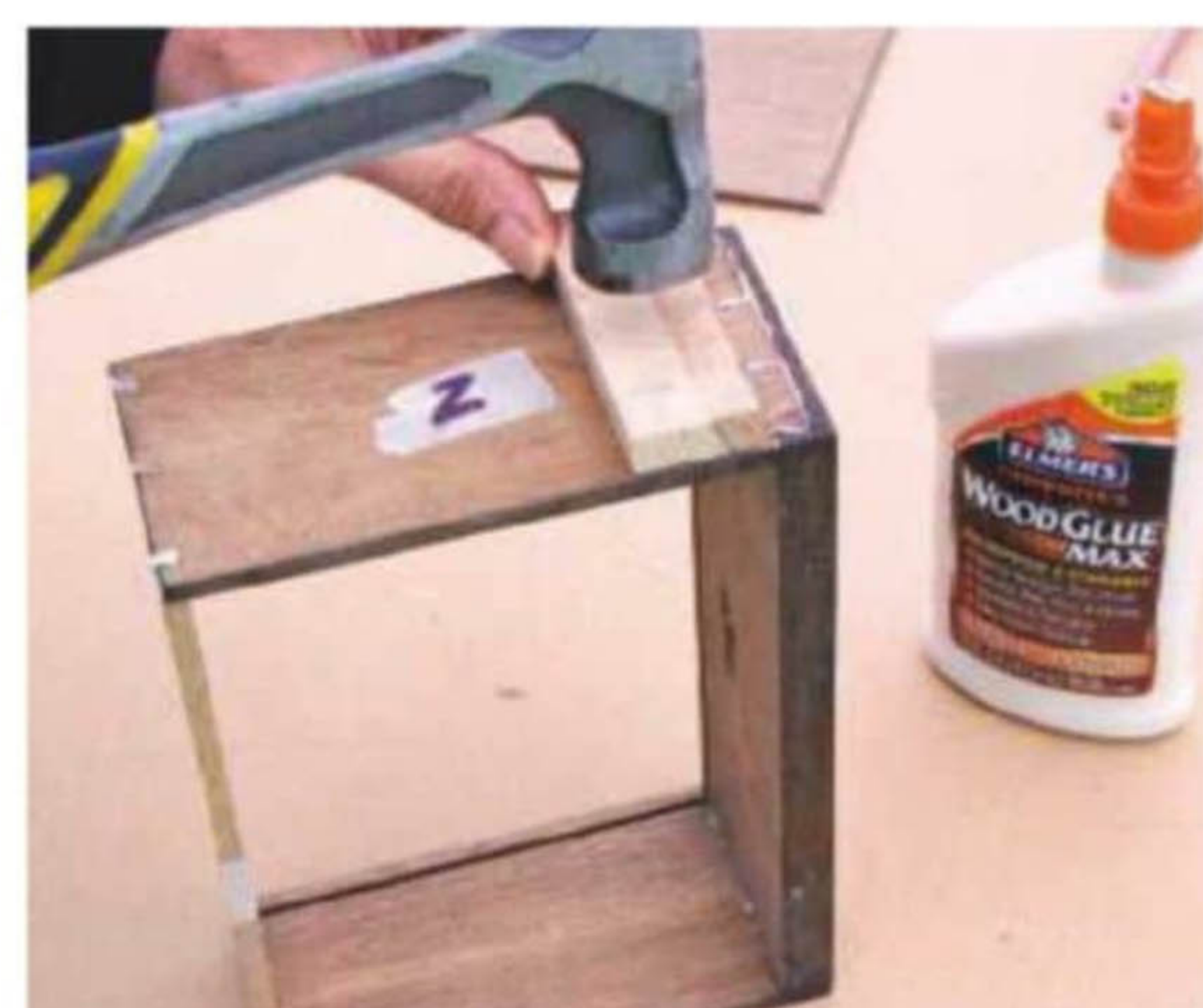
30 Apply PVA glue to dovetails and tap components gently together; add bottom to drawer
