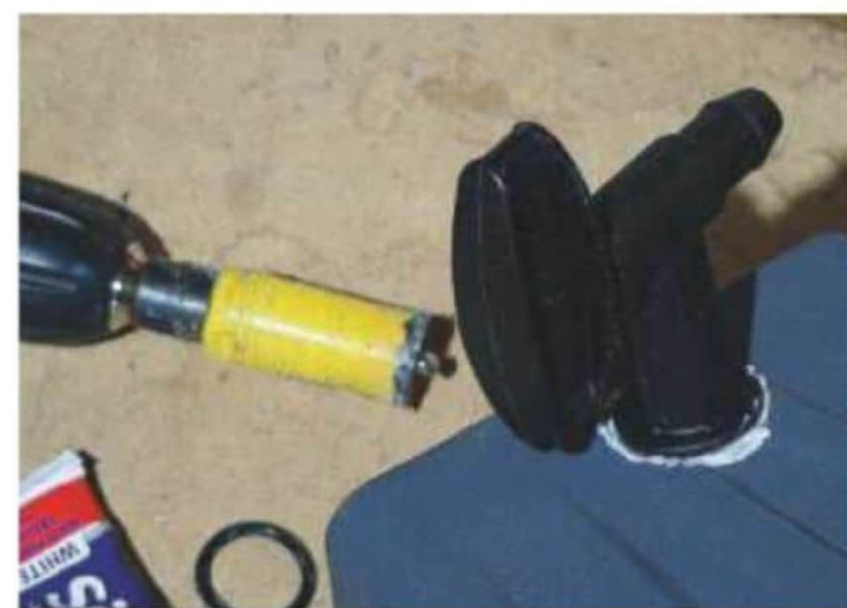
17 Drainage tap installed
