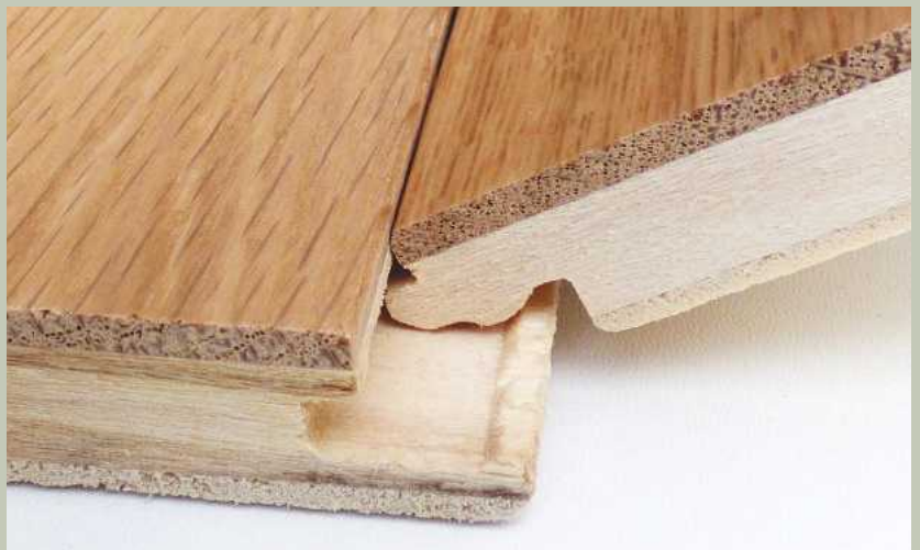
Click fit boards are faster to lay as they don't need gluing together
