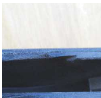
Damage to the crown guard when it twisted
