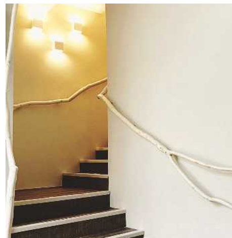
Locally sourced ash timber shaped into bespoke staircase handrails
