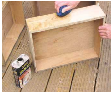
11 Lightly sand, then stain wood to restore the colour; to check this, test on the back of a drawer first
