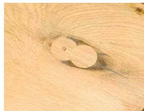
22 The two infill discs in place
