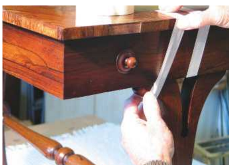
18 Masking tape is ideal for holding things in place
