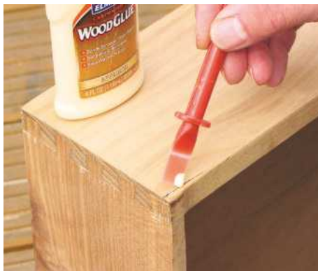
7 Glue and cramp any split drawer components or edges that are loose; sand once the glue has dried
