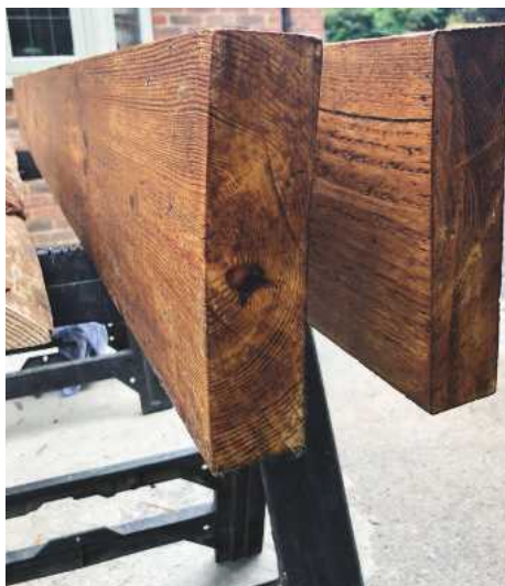
7 8x2 joists after receiving a second coat of wax
