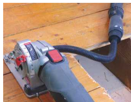
Using the Project Vac connected to a Skilsaw Multi when cutting through floorboards was an ideal test, as small saw tools like this can throw out a surprising amount of sawdust
