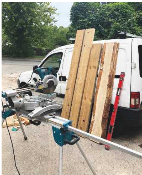
3 All lengths cut to size ready for the next step
