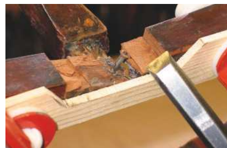
39 Making recesses for the new wood
