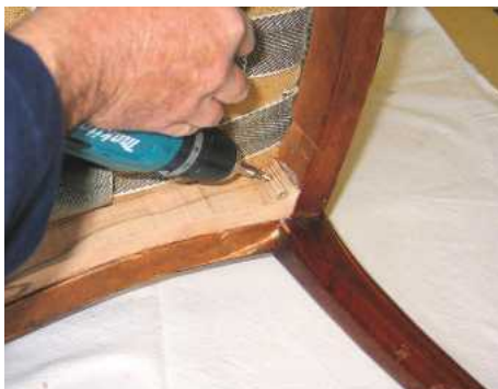
45 Fixing the extra piece in place
