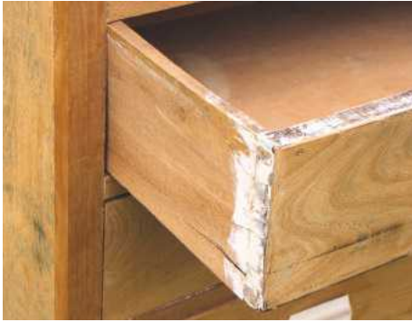
3 Some drawers may be worse than others; although these fronts are dovetailed, backs are only nailed to sides
