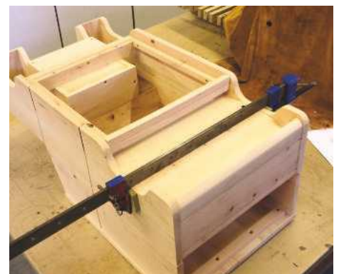
12 The bottom, flat platforms are next
