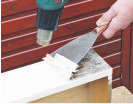
4 A heat gun used with shave hook or stripping knife is the fastest way to remove several layers of paint
