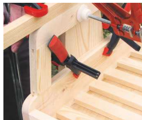
21 Cramp the tapered sides to the lower box to keep everything aligned while the glue dries
