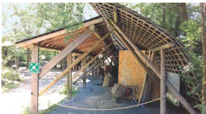
7 Another demonstration area showing use of roundwood laths and shingles. This area is used for the 'wet trades' courses on hempcrete and suchlike
