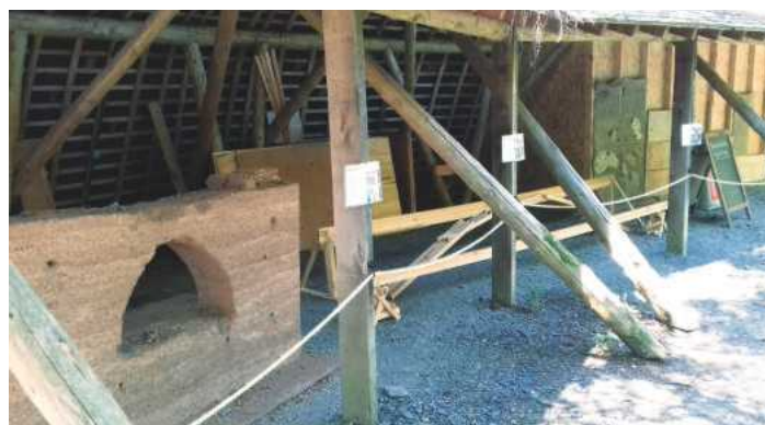
8 An example of a rammed earth arch. This is a truly sustainable method of building, but hard work. The lecture hall at CAT is the largest rammed earth building in the UK
