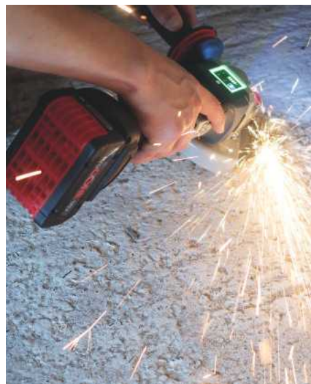
Cutting a metal pipe from the workshop floor
