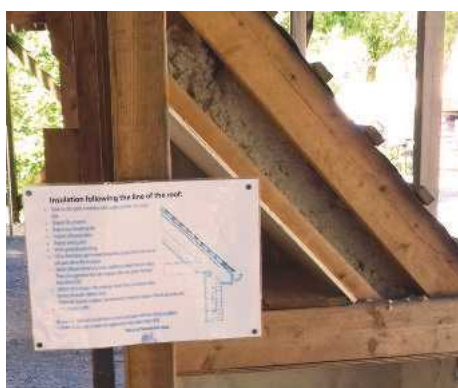
12 ... where to put the insulation and why...
