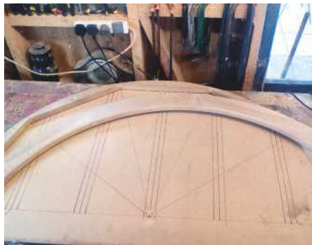
5 &amp; 6 Cutting the curves
