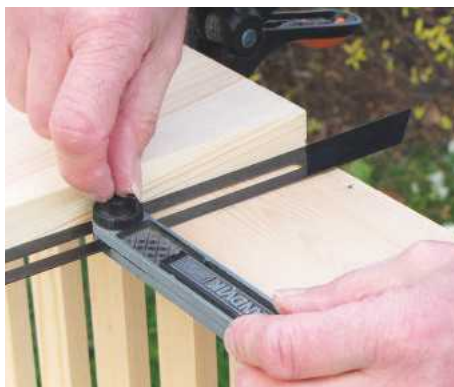
17 Set a sliding bevel to the angle formed by the taper. Upper side components are cut to match
