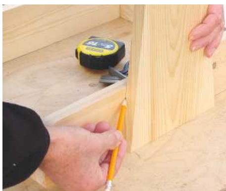
13 Hold the tapered sides against the box and mark centrally to determine the inside screw positions
