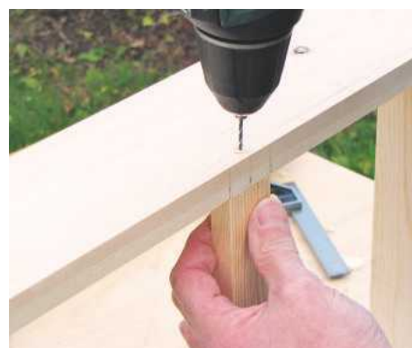
15 Each slat is glued and nailed in place. Drill pilot holes to prevent the wood from splitting
