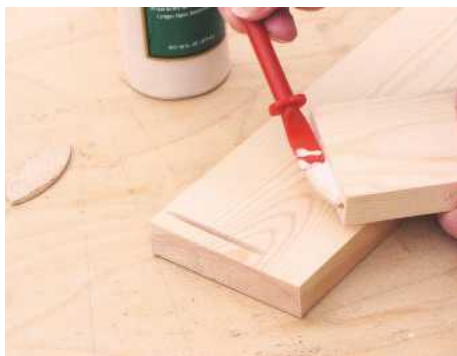
4 Sand inner faces of the sides and ends. Spread the biscuits with PVA glue and insert them into the slots
