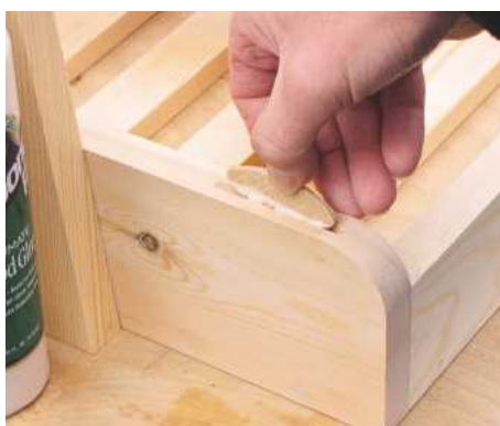
20 Cut matching slots in the top edges of the lower sides, then glue the upper rails to the lower box
