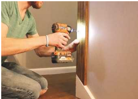
10 Attaching one of the extra boards to the wall once cut to fit the space....
