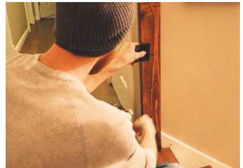
12 Hanging one of the hinges
