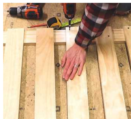
6 Pre-drilling and adding screws at the locations where the boards overlap
