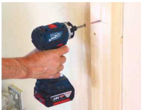
12 Drill screw clearance holes in the timber and mark the wall. Drill masonry and insert plastic plugs, then screw the stud into place
