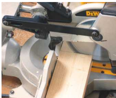
16 Measure each stud position separately as the ceiling may not be flat. Cut studs to length with a mitre saw for speed and accuracy
