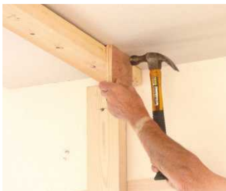
15 Cut the head plate to length and tap it into place. You may need to force this upwards with a stud if the ceiling is bowed
