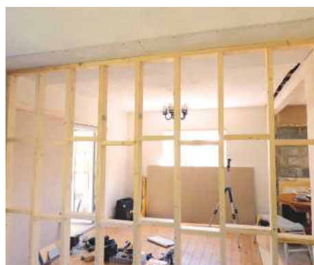
23 Noggins are easier to nail if they are staggered, rather than in-line. The finished partition should look something like this
