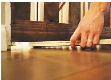
13 Adding a board under the gate to lift it 20mm off the ground
