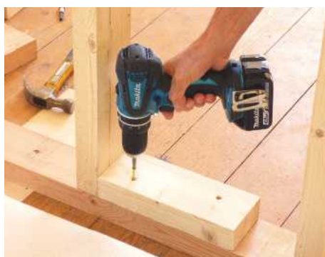
19 To prevent studs shifting sideways when nailing them to the floor plate, screw blocks temporarily to stop any movement
