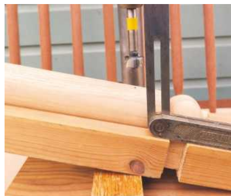
15 Drilling arms using an 18mm sawtooth bit
