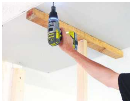
14 If overboarding the ceiling is required (to cover artex), screw 9.5mm plasterboard sheets to the joists above the studwork
