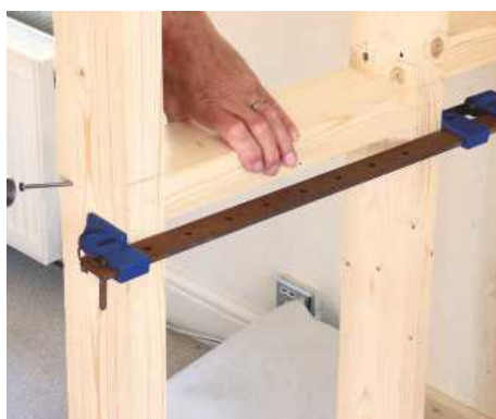
22 Measure each noggin and saw these to length. A cramp across each pair of studs prevents them slipping during nailing
