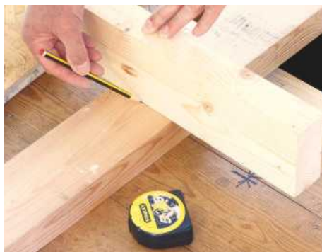
13 Mark out equal positions for the remaining studs, checking that full plasterboard sheets will join midway on the relevant timbers
