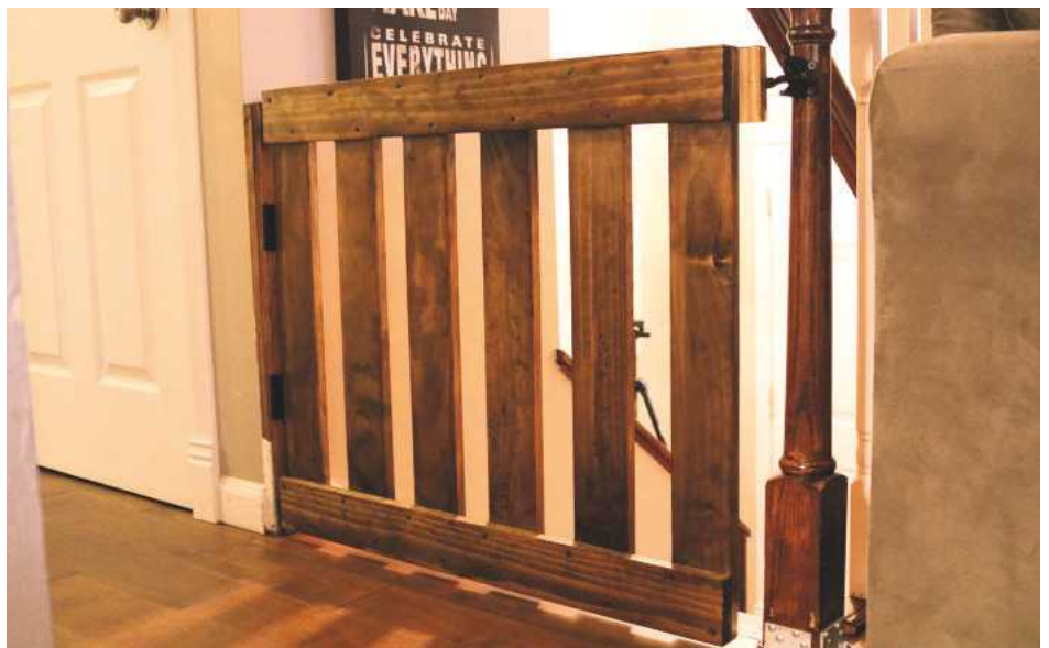
15 The completed baby gate in situ
