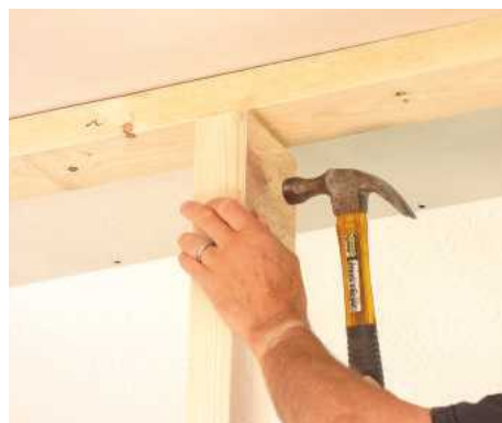
17 Drill and screw the head plate to joists or noggins above. Fix a stud at the far end, then cut and wedge remaining studs in place
