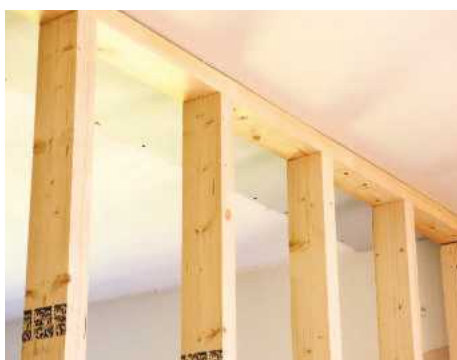
18 Check the stud centres coincide with the width of a plasterboard sheet. If not, tap them until they're spaced evenly
