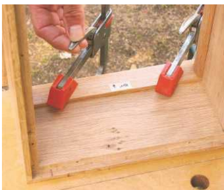
38 The door stop is simply 12mm wide strips of oak glued around the inside. Fit these with the door in place
