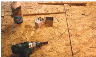
8 OSB back stiffened with additional fillets
