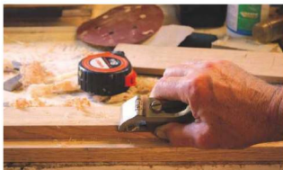
9 Sharp arrises removed from doorstep
