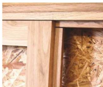
19 Cover strip fastened to back of left-hand door to seal gap between double doors
