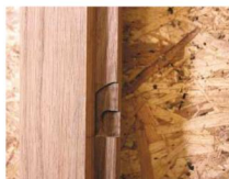
21 Cut-outs in door cover strip to accommodate the lock
