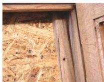
22 Batten fastened to inside of cabinet to help with fitting notice board in position
