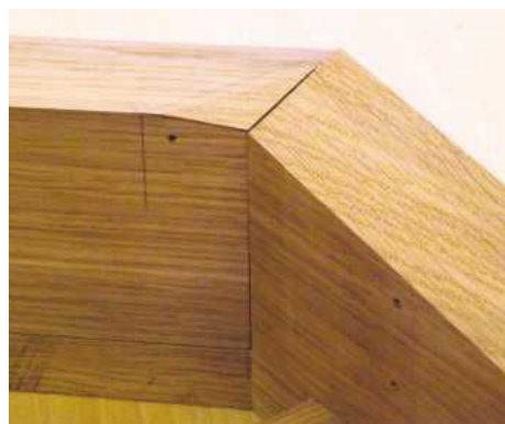
19 East and North-East close to completion
