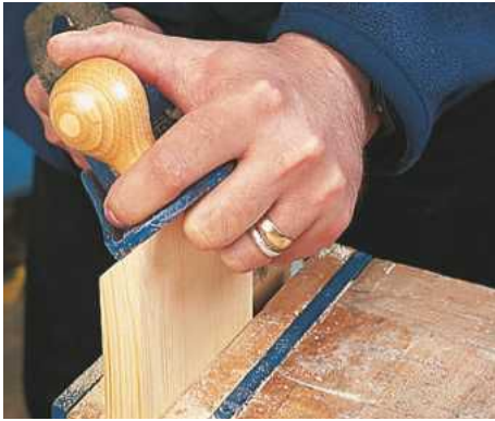
Sawn mitres may need planing to fit
