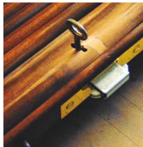
10 Once the glue has set, the plug's trimmed back ready for staining, etc.
