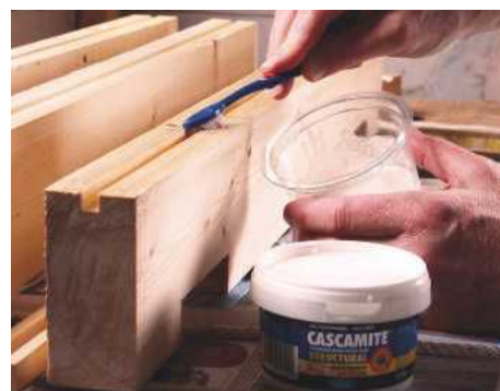
25 Applying Cascamite by toothbrush
