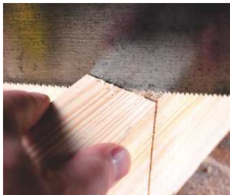
7 ... and sawing from all sides to make a square cut
