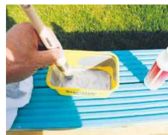
A sparse amount is needed; a small squirt of Extender allows for a longer working time
