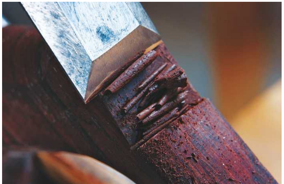
20 Chiselling a bed to receive the repair piece
