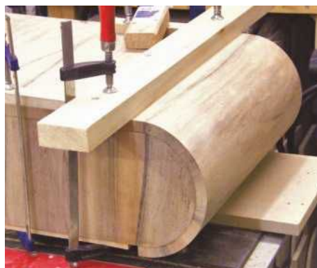
23 When gluing the shelf in place use a batten to keep the shelf flat with the curve
