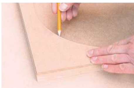
10 When the template is accurate, lay it on the MDF panel and draw around the arch. Flip and repeat for the opposite side
