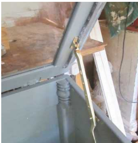
15 Strips of glued-on foam rubber cut from packaging should protect little fingers if the children drop the lid on themselves by accident
