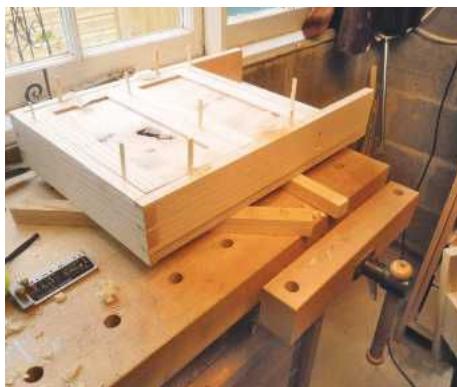
9 After having been shot to fit, the doors are wedged in place while the hinge housings and door knob positions are marked
