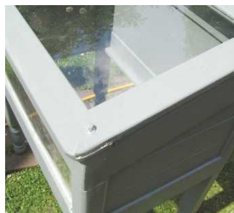
14 Reassembly with the glass is simple. The lower side of the cold frame was panelled with acrylic, not wood, to let in more light safely
