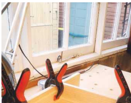
8 To give the doors something to close onto, without the complication of cutting rebates, 6mm-thick linings were glued in
