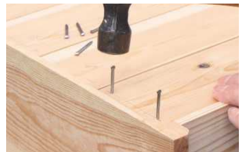
29 Cut the matchboard to length and saw outer boards to width if needed. Pre-drill and nail into the rebates
