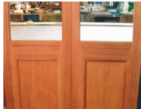
7 The inner face of the doors; the ovolo moulding is a replica of mouldings on the existing shutters
