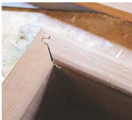
6 ... though the mating faces did need some cleaning up
