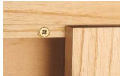
16 ... holding against a small screw in the door stop
