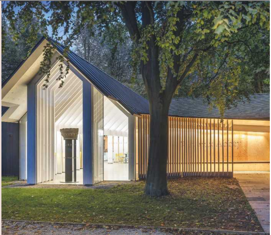
The Rievaulx Abbey Visitor Centre & Museum creates an abstract, numinous space using timber as an expressed structure
