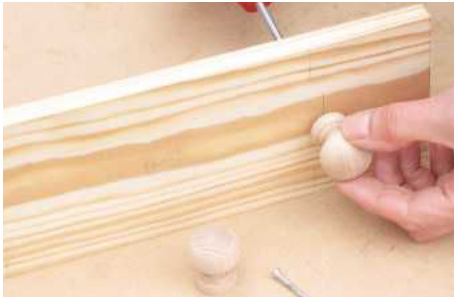
21 Mark and drill the drawer front for knobs before gluing up. Counterbore the rear screw heads
