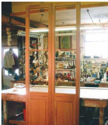
8 The outward face of the doors; the panels are flush, surrounded by a captive bead – typical of mid-Georgian work
