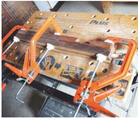
16 The new runner strips were glued into place
