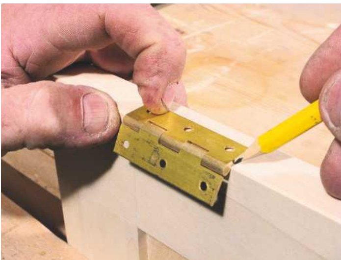
3 Place the hinges in position and lightly mark out using a pencil...
