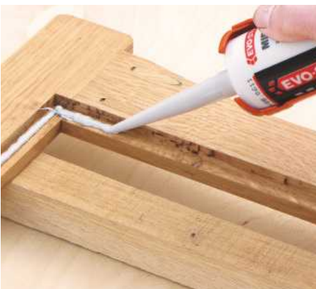
23 Apply a thick bead of mirror fixing silicone around the glass rebate. Don't skimp on this
