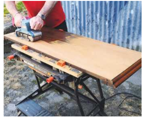
17 Using a belt sander, with care, the worst of the old surface finish was taken off
