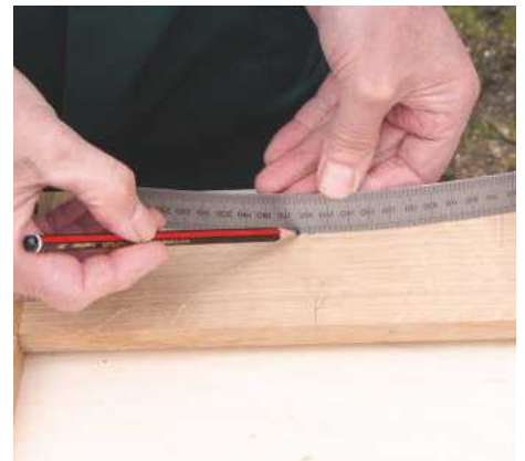
8 Draw a curve on the bottom rail by springing a steel rule between two offcuts cramped in place
