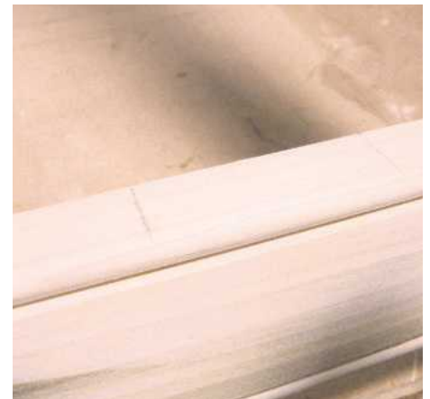
13 Lightly square the marks across the frame using a pencil...
