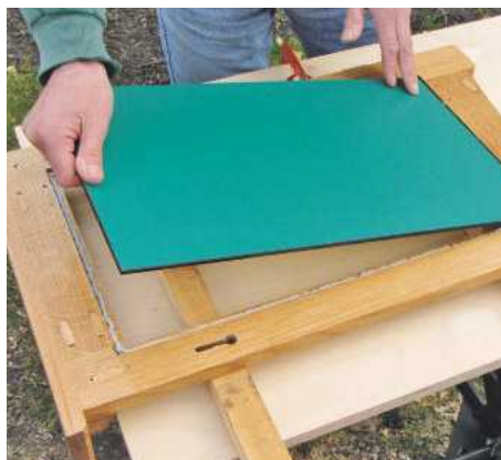
24 Lower the glass into the rebate and gently apply pressure all the way around the edge
