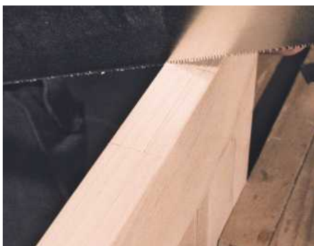
7 Make a series of cuts into the waste using a saw, sawing slightly shy of the knife lines
