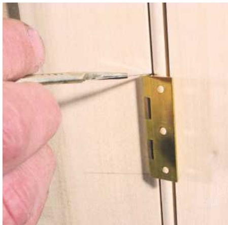
12 Use a scalpel or marking knife to mark the hinge positions on the edge of the frame
