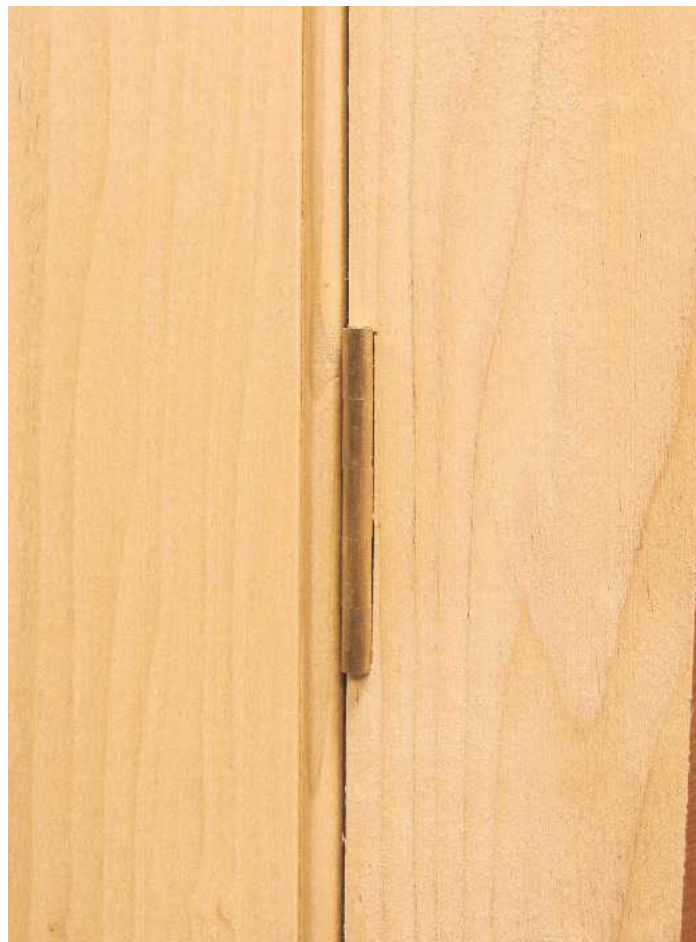
19 The hinge could have been recessed into the frame bead, but here the vertical lines are uninterrupted
