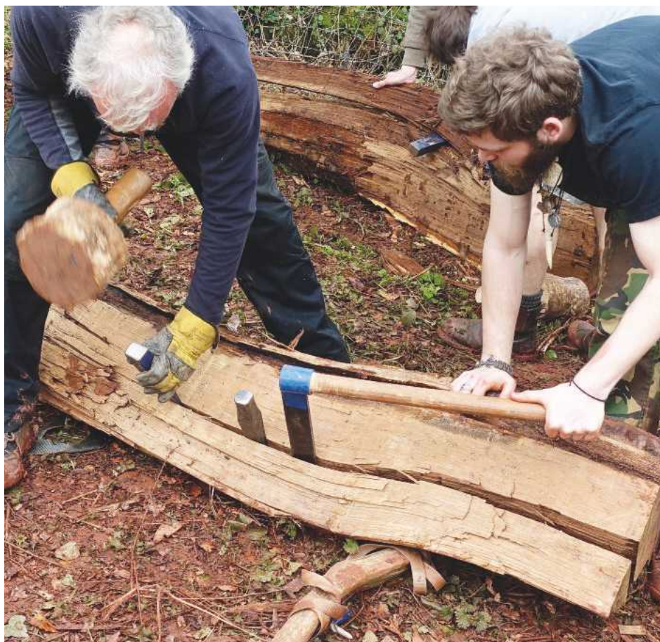
A baulk being opened up with froe and wedges
