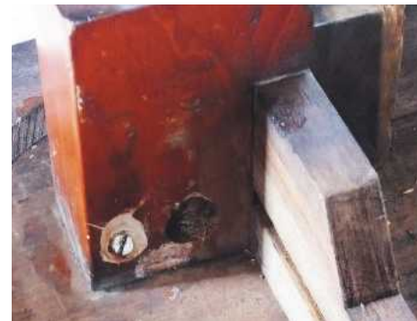
11 Back in place this leg had a new, pocketed screw driven in to help hold it along with the re-glued mortise & tenoned rail
