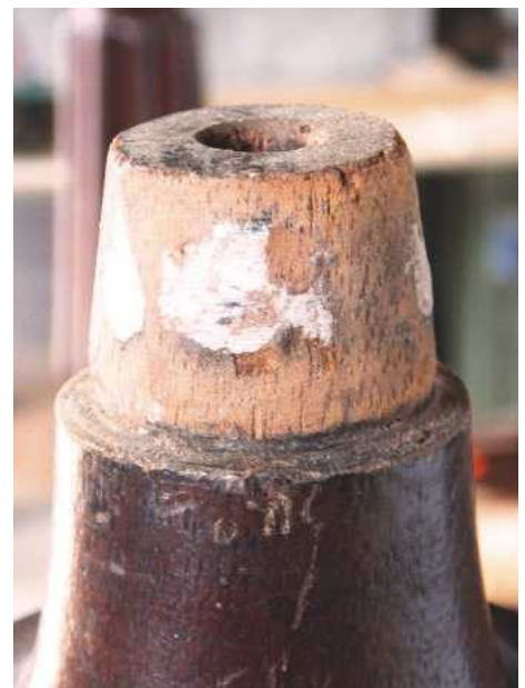
8 One of the first jobs I had to do was to fill up the old screw cavities
