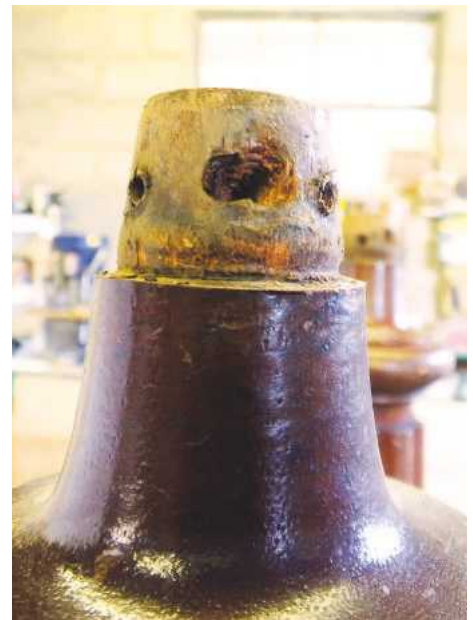
7 The old screw fixing holes had little real wood left
