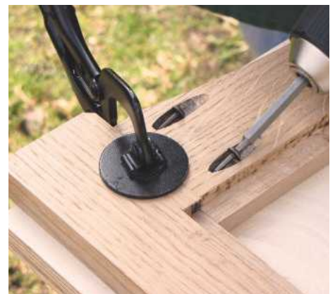
11 Brush on PVA glue, clamp to a flat surface and screw the rails and stiles together
