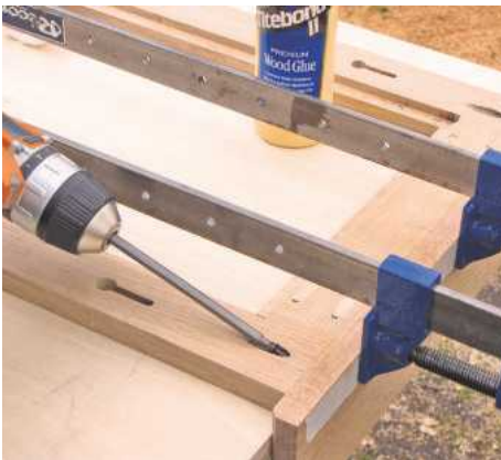
18 You can then apply glue to the top of the frame and clamp the shelf in place. Fix with pocket screws or biscuits
