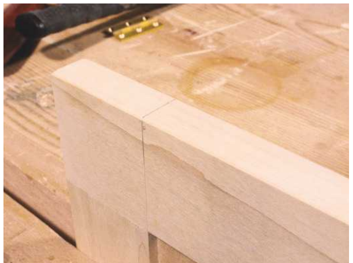
4 ... then, again lightly, square the pencil lines across the door edge and face
