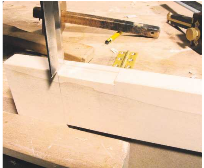
11 The last task is to locate the chisel in the knife lines and remove the sliver left by the saw
