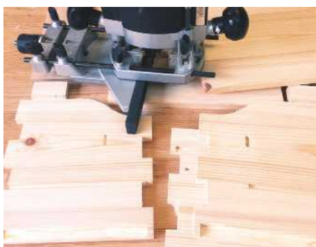
7 Some careful router work produced the necessary grooves and rebates in all the components
