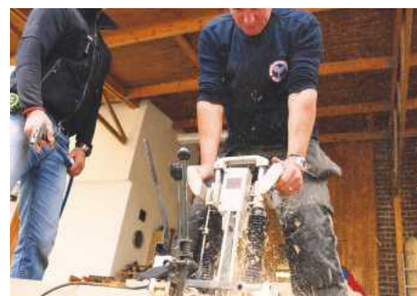
Cutting a mortise with the portable mortiser
