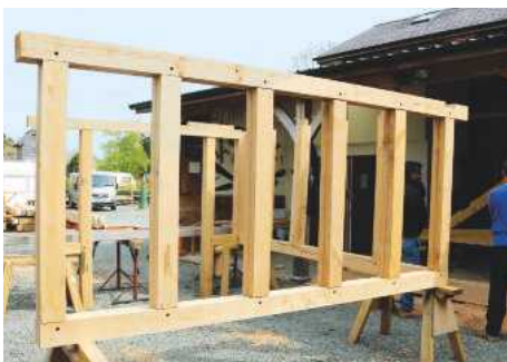
Two sides and half an end ready for the main beam
