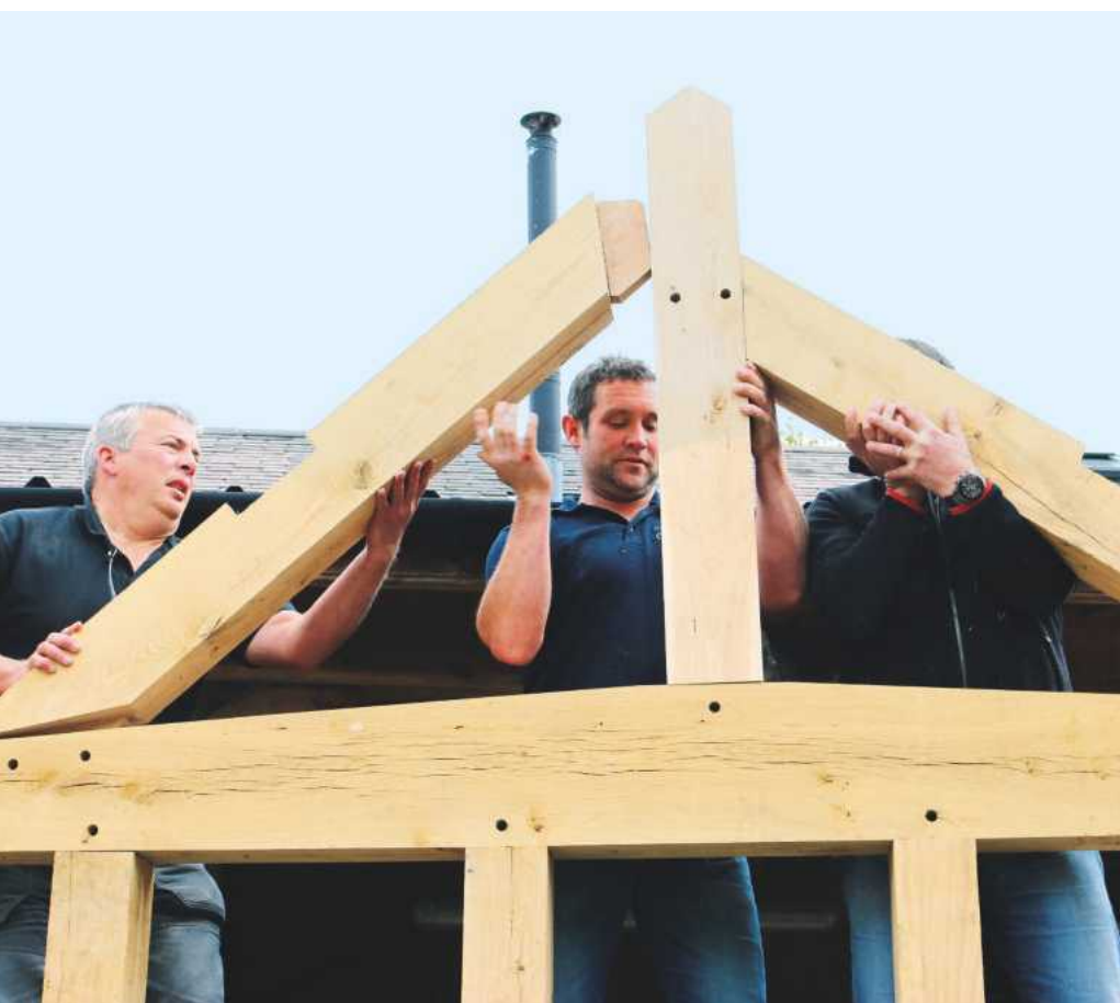
Trying the fit – notice how the tenon is cut to allow it to fit at an angle
