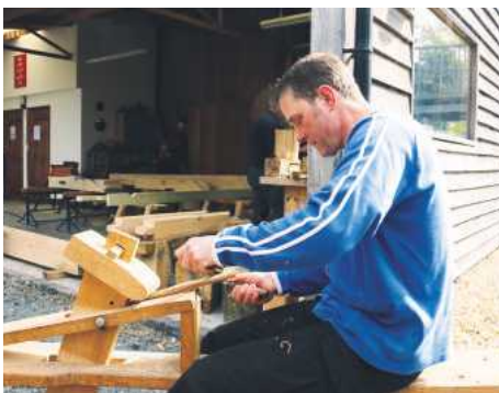
Using a drawknife to make pegs for joints
