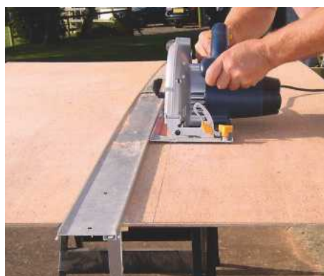
1 I cut the ply with a circular saw...
