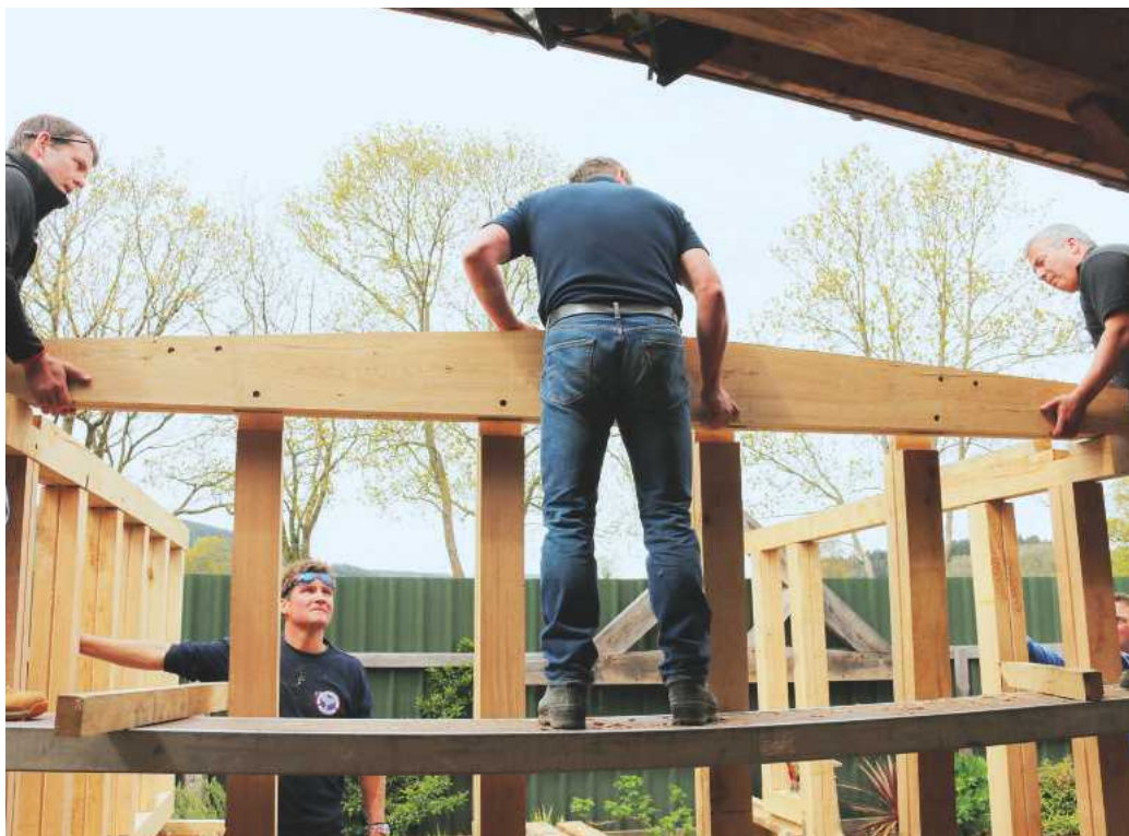
Fitting the main beam
