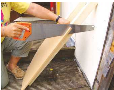
4 Leaning the work against a couple of timbers makes it easier to rip thin boards
