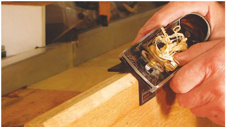
11 A chamfer was formed on the drip board...
