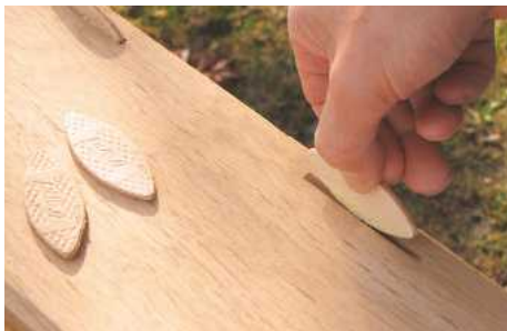
13 Use No.20 biscuits for fixing the upper shelf to the rear panel. This size is also used for the end pieces
