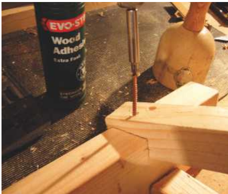
7 Apply glue then pre-drill and countersink to allow for 75mm screws
