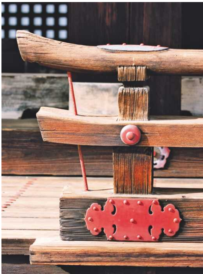
An architectural detail from the Imperial Palace in Kyoto, Japan
