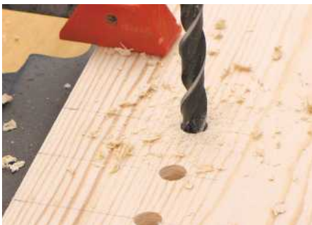
11 Mark support spacings and drill 10mm holes for the collars. Three rows mean you can alter the height of the shelf
