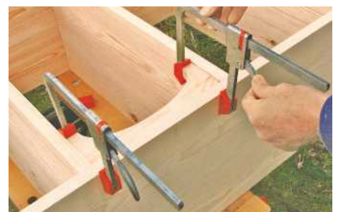
18 Fit a decorative apron under the top panel in the centre. Cut out the arch with a jigsaw and clean up
