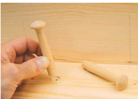
23 A row of Shaker pegs are glued into shallow holes in the panel along the base of the unit
