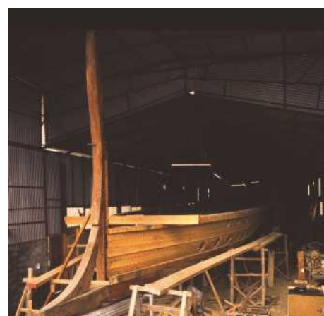
Setting out the deck for the upper level of oars
