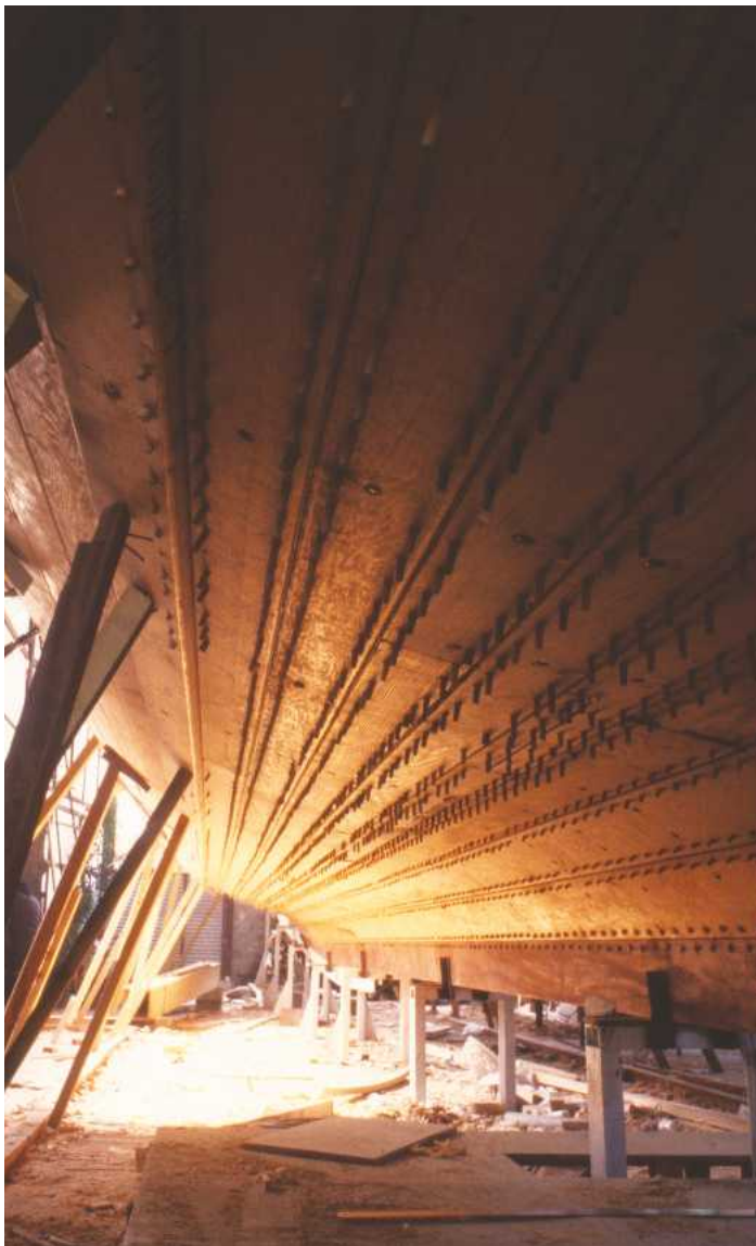
Detail of bottom planks as work progresses
