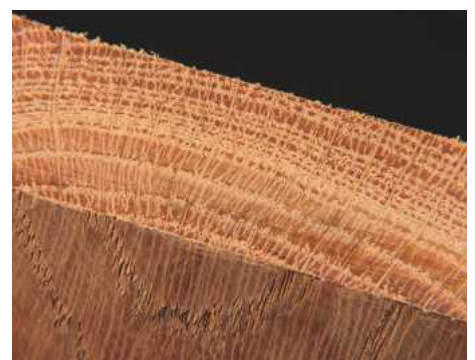
17 End-grain of a reconverted elm board
