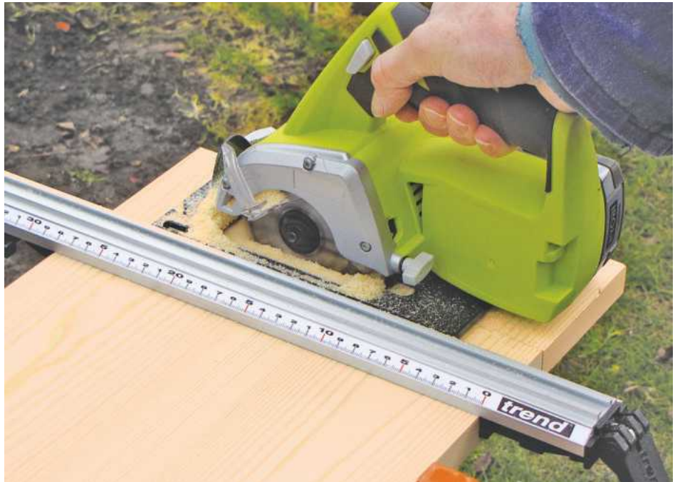
19 Shelves are made shallower to allow for door thickness. Cut boards to length and plane the ends square
