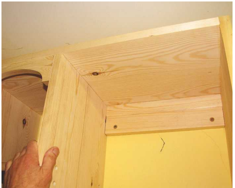
24 With cleats fixed under the top panel, lift the unit so they locate over those screwed to the wall
