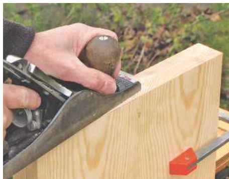
3 Saw the side panels to length, then clamp together and plane to width. Plane both ends square
