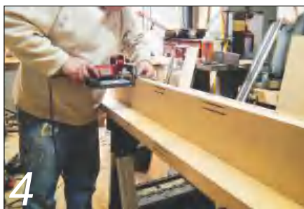
4 Double rows of No.6 biscuits are used on the main boards
