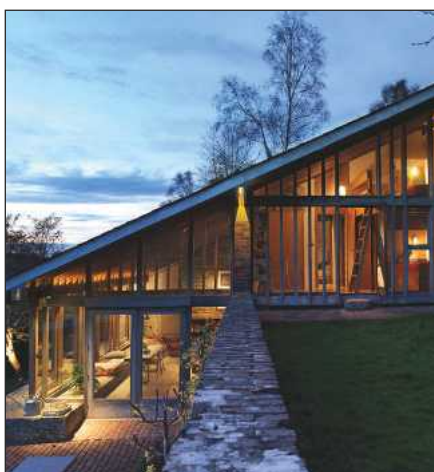
Ansty Plum has undergone a retrofit and studio extension
