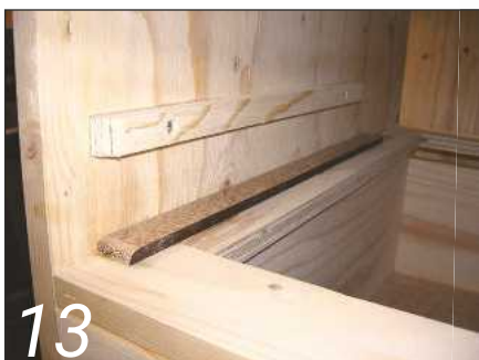
Ply guides and waxed hardwood 'wear' strips should make the drawers run smoothly
