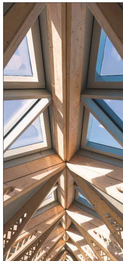
The roof is naturally illuminated by triangular roof lights and is supported by lightweight timber lattice beams
