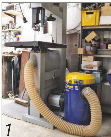
The dust extractor is linked into the bandsaw's controls so that it starts automatically whenever the bandsaw is switched on. This is an ideal arrangement
