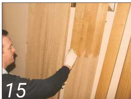
15 Once sanded, all the parts were finished with two coats of Osmo Polyx oil
