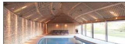
Flitched feature trusses support the roof over the swimming pool
