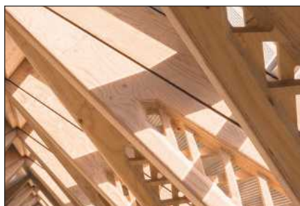
The lattice beam structure is made using Nordic spruce
