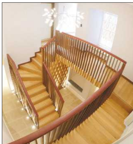
The spindles of the staircase are cut with arcs of varying sizes to create an organic flow
