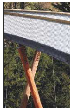
Siberian larch is used for the columns due to its tighter grain and higher strength-to-weight ratio
