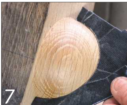
... and keep offering up a template to ensure accuracy
