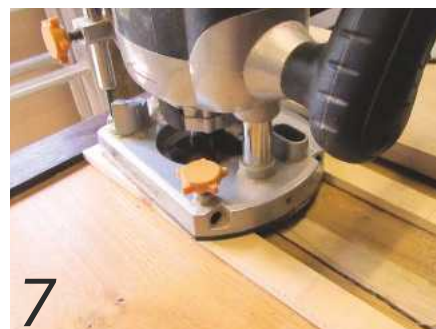
7 Rather than cut out the whole of the damaged area, I cut a shallow trench over it. The block beyond the router acted as a fence; the pine pieces beneath allowed me to cut right up to the sides...
