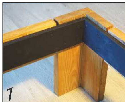
1 Inside corner detail. The screws through the matt black ply are plainly seen
