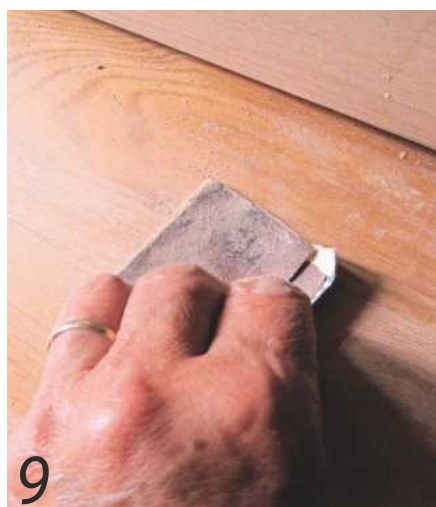
9 ... and a few shims of veneer lifted the new slice to the correct level for final sanding
