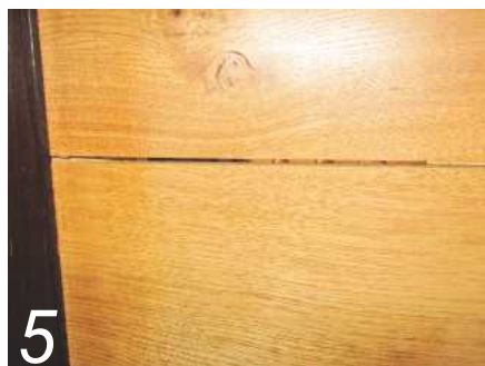
5 A slim split of constant width turned out to be just wide enough to take an edge-on slice of matching wood
