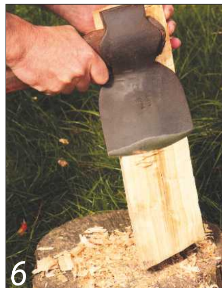
First flattening of the split surface with the side axe...
