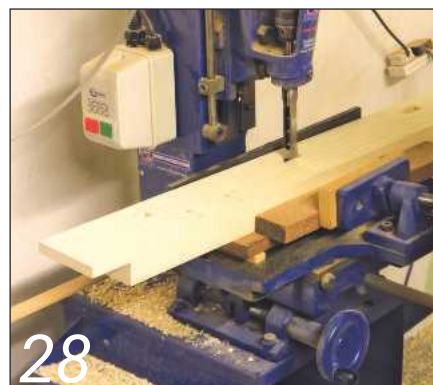
28 The mortise holes are slightly canted by using packing
