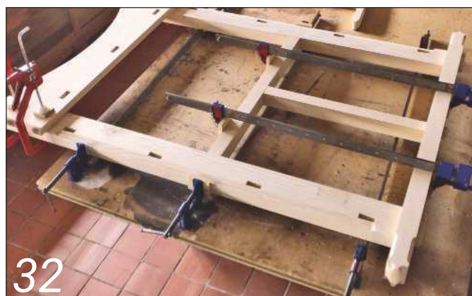
32 With all the joints cut, the sub frame is glued up
