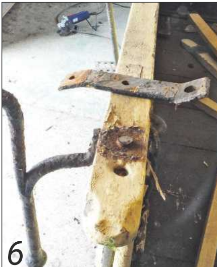
6 These brackets had to be cut off
