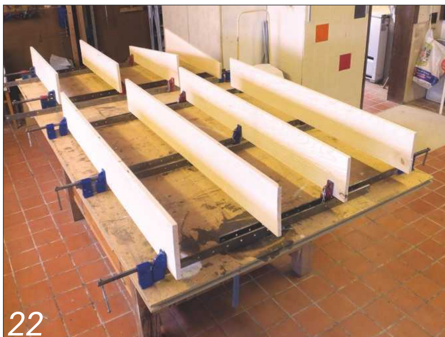
22 The four panels are ready for gluing
