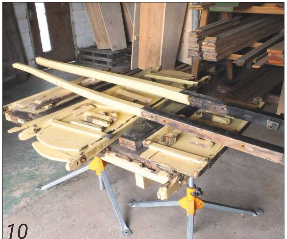
10 Once apart, this is what the woodwork looked like
