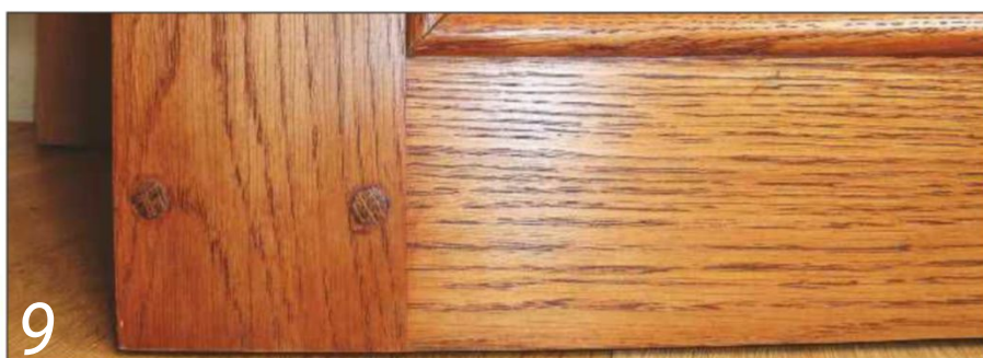
9 The dowels used for filling the fixing holes were left slightly proud and rounded over to give an authentic look to the job
