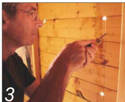
Joining up the holes with the pad saw
