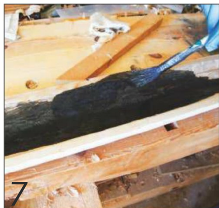
7 The thinness of the graphite and shellac mixture meant that four coats were required...
