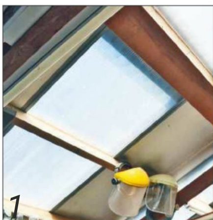
My workshop features a well insulated pitched roof with panels, which emit natural light
