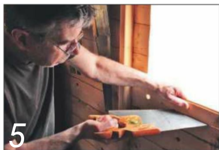
5 Ripping through the bottom plank
