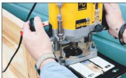
A heavy-duty router is needed to rout out the lock case, or you can drill and chisel if needed
