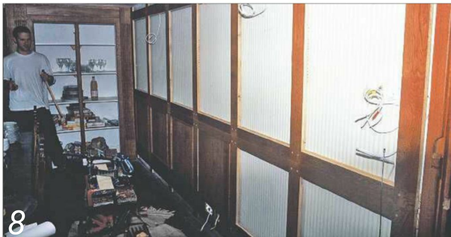
8 On site the frames were fitted into place before slotting in the panels and fitting the mouldings
