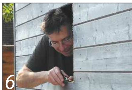
6 Tidying an edge with the apron plane
