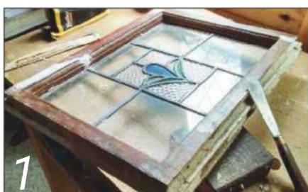
Victorian leadlights undergoing repairs
