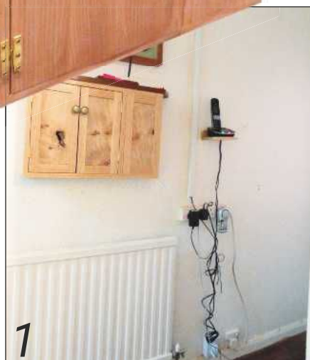
1 My brief for this project was to hide a selection of untidy, long-standing ‘temporary’ electrics in our hallway
