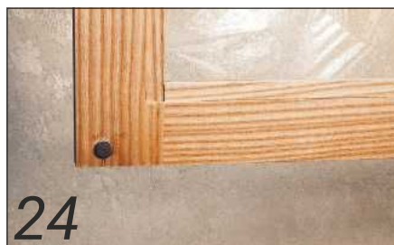
24 The doors are held closed with rare-earth magnets
