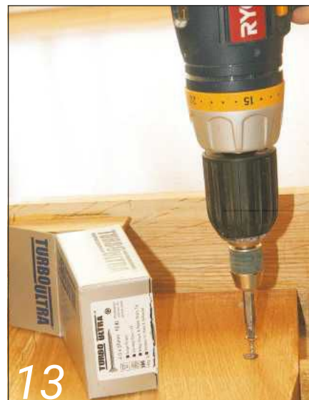
13 French cleats make the mantelpiece easy to remove for access to wiring
