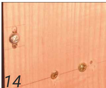
14 Before adding shelves 4 and 5, cut the expansion slots for the screws that will secure the cubby hole front panel
