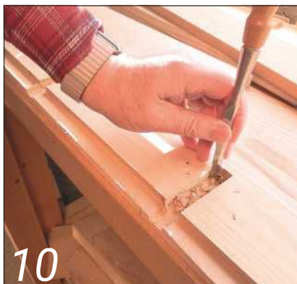
10 Squaring up the routed housings is easily accomplished with a sharp chisel
