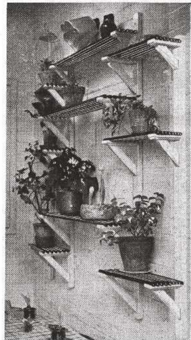
FIG. 1. DESIGN WHICH BREAKS AWAY FROM THE CONVENTIONAL. Instead of solid shelves a series of slats or beads is fitted, giving a light appearance. These slats are painted black and look well against the cream paint of the main framing.
