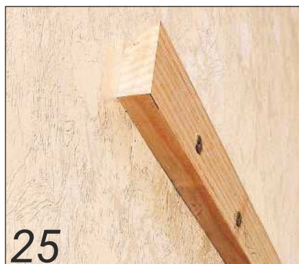
25 A corresponding batten on the wall serves as a hook
