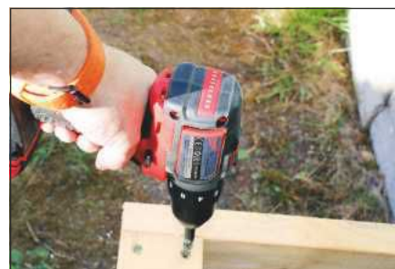
Constructing some decking with 100 x 6mm screws was a breeze
