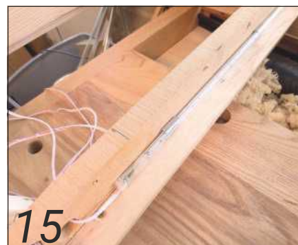
15 Attached to the back of 10mm-thick strips in the display section are the baffles that hide the lighting strips
