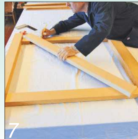
7 The brace top and bottom rail mortise holes have been marked and now the shoulder slope of the tenons is taken straight off the dry assembly
