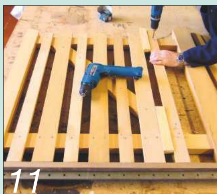
11 Finally, the pales or 'pickets' are fixed to the gate's frame
