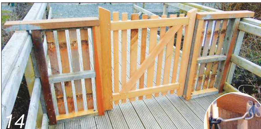
14 The completed gate with its added hand-made touches
