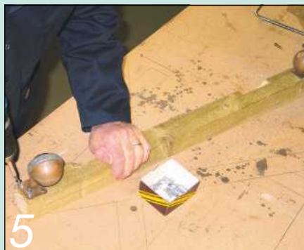
5 Fit the castors to the lower brace before fixing it onto the leg assembly
