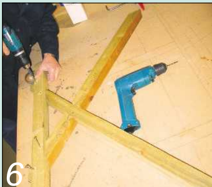
6 The brace with castors attached is screwed and glued on
