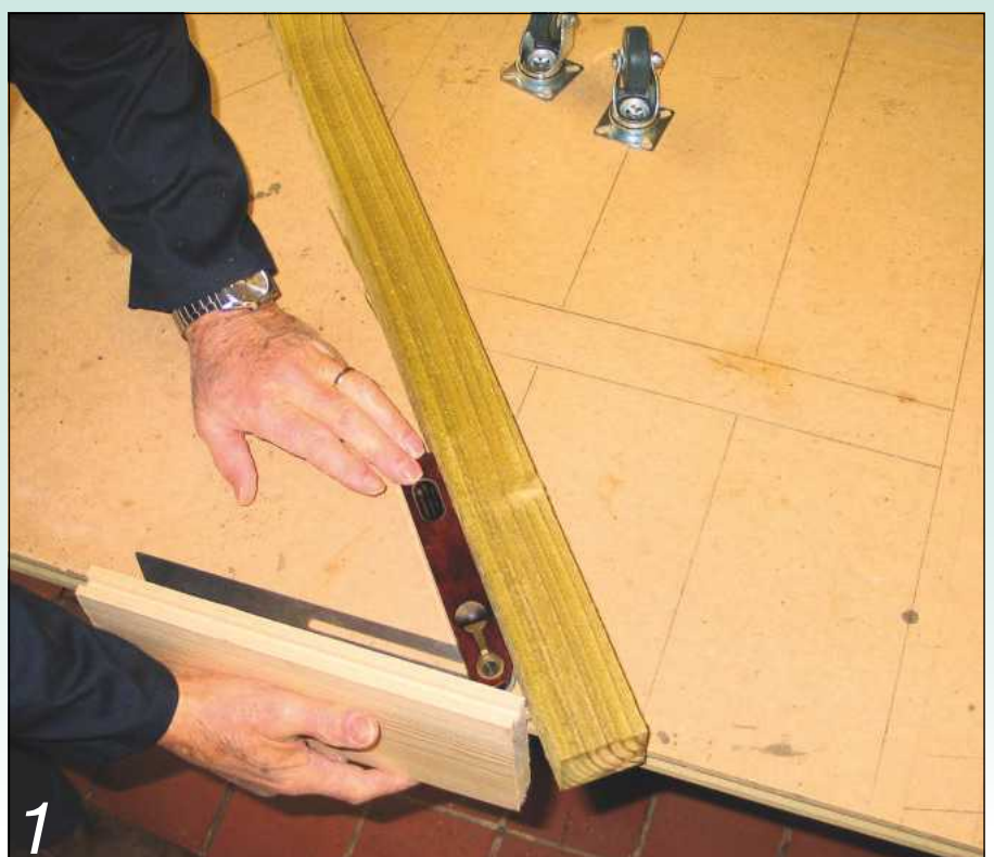
1 Angles can be taken straight off the full-size drawing
