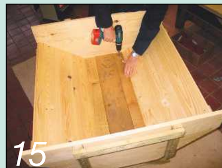
15 The bottom boards are then fitted
