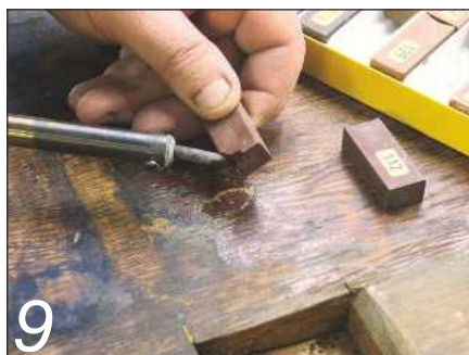
9 Melt hard wax into the hole...
