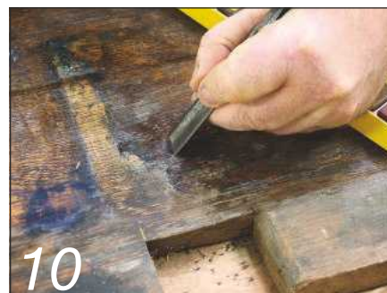
10 ... and scrape away the excess
