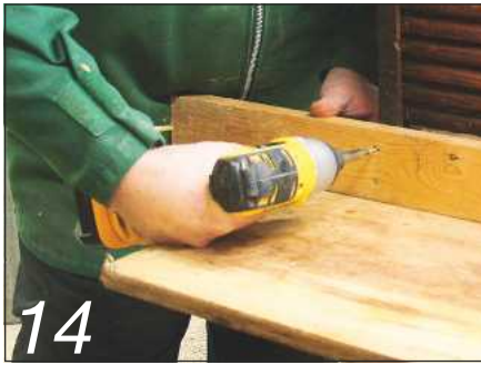
14 A temporary brace kept the sides in the correct place...
