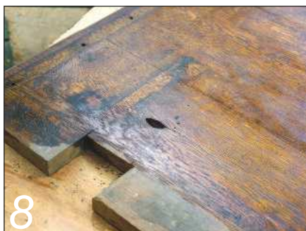
8 I don't know how this hole came about, but it needed filling
