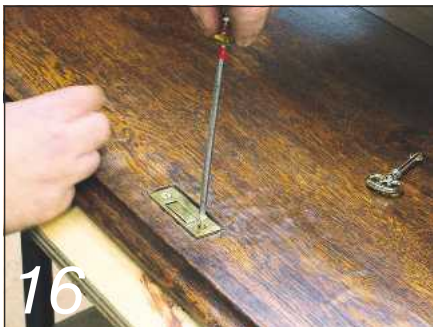
16 The strike plate was installed next...
