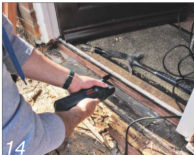
14 After removing the water bar for re-use, the remainder of the cill is removed
