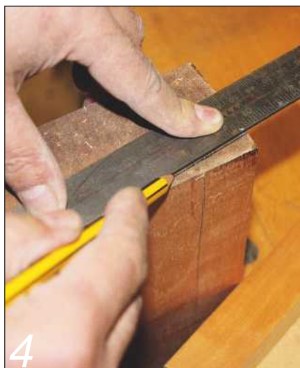
4 Determine how much of a bevel you need and mark it up on the cill
