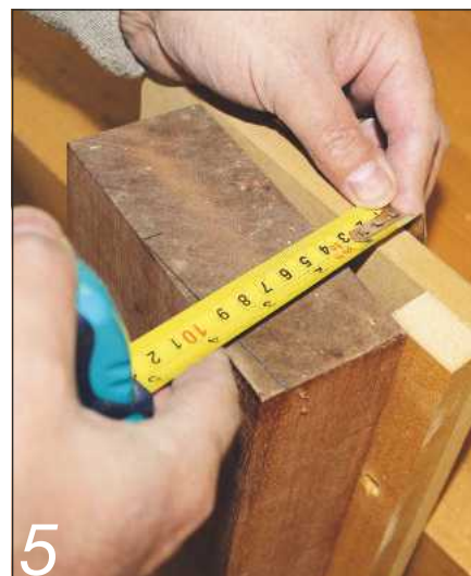
5 By moving the cill further along the batten, the pitch alters. Move it until it's parallel and mark the jig
