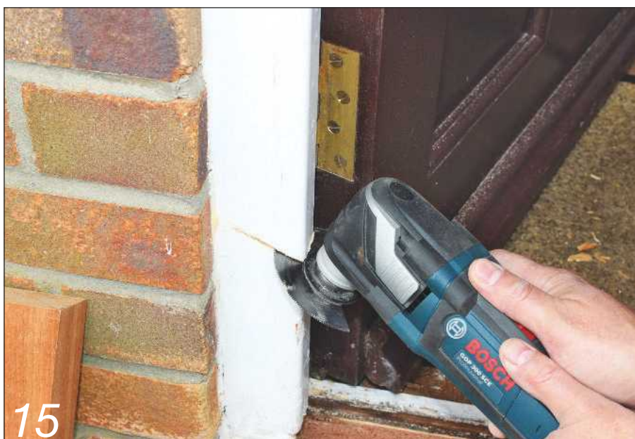
15 The rotten jamb is cut away next. A multi-tool is worth its weight in gold here!
