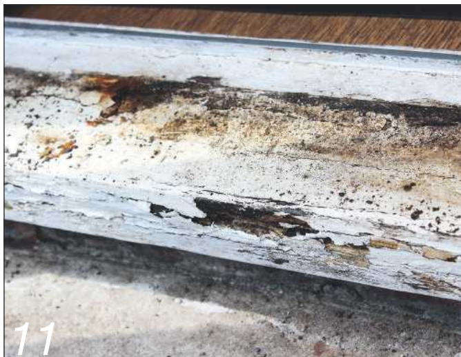
11 After the protection plate is off, the extent of the rot can be seen
