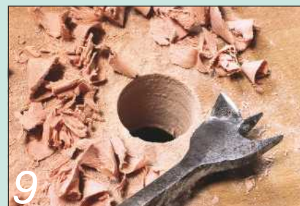
First of three holes completed
