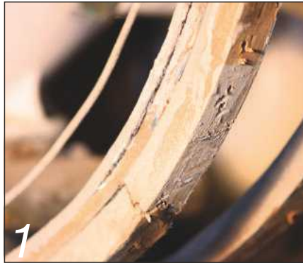
1 The yacht's original timbers had started to crack as her hull shape deteriorated
