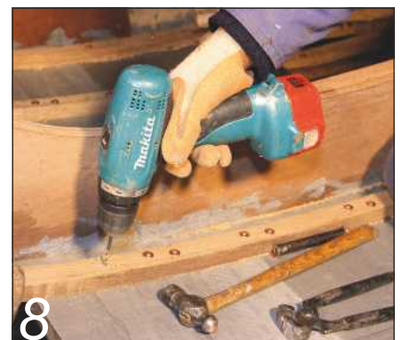
8 The nail holes are staggered to avoid any risk of splitting the new timber
