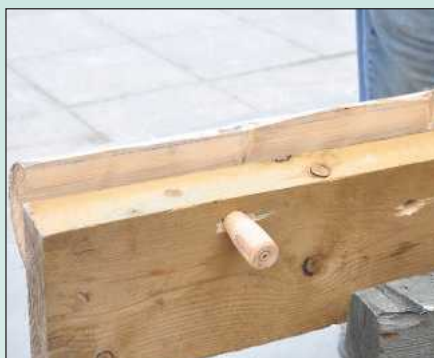
The stile was then repositioned on pegs against the face of the bench so the edges could be planed true
