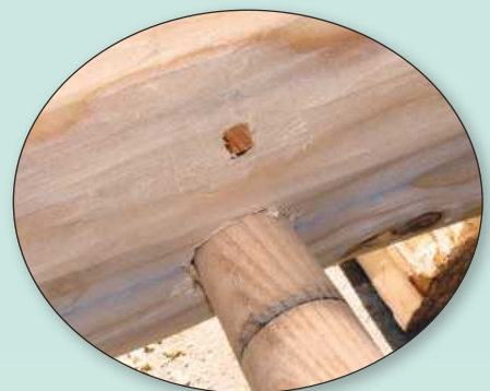
Angled holes were drilled through the stile into each rung (left), ready for a wooden trennel to be driven in and trimmed off (above)
