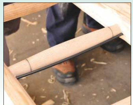
Careful angling of the drilled holes forces each tie rod to follow the profile of the run for maximum support
