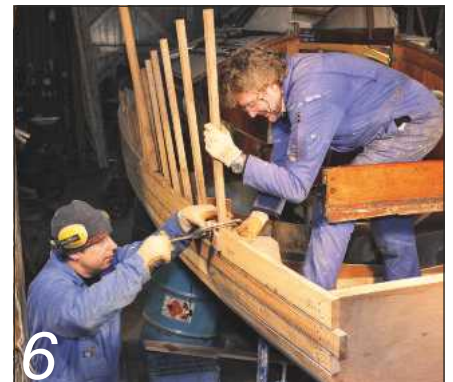
6 A clamp is fitted at the turn of the bilge to hold the timber securely in place
