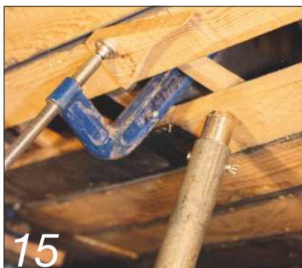
15 This particular dolly consists of a metal pole with a heavy weight on the end
