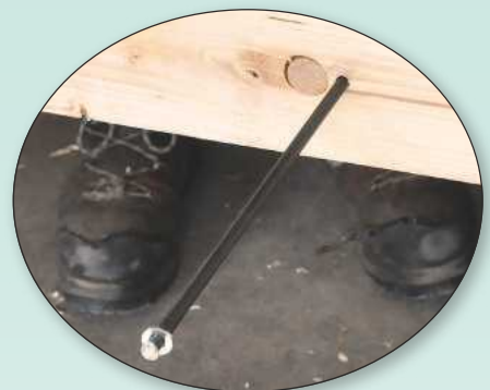
Each tie rod is fed through its pre-drilled holes (above), and the free end is then hammered over to lock it in place (left)
