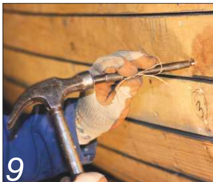
9 Dean then uses a centre punch to drive the nail fully into the countersunk hole
