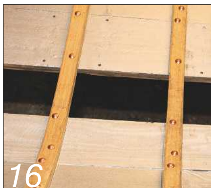
16 The last of the steamed timbers have now been fixed securely in place
