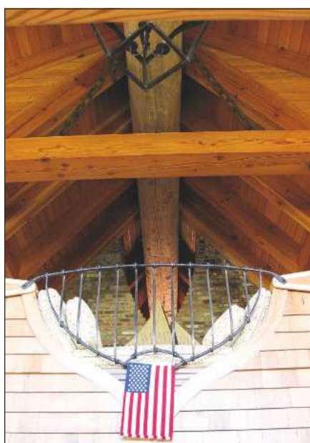
The Beam is currently playing both a starring and a (roof) supporting role
