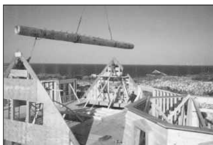
...and slowly lowered inch by inch towards the huge gable end walls of the main house
