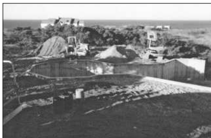
At the house site, the massive concrete coffer dam foundations went down...
