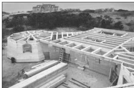
...and the house began to take shape. There's no timber shortage in the USA!
