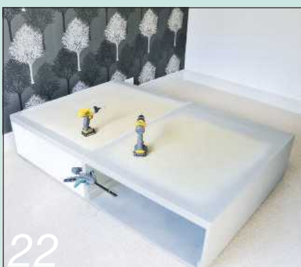
22 The two base pods were clamped together and joined with cabinet connector bolts
