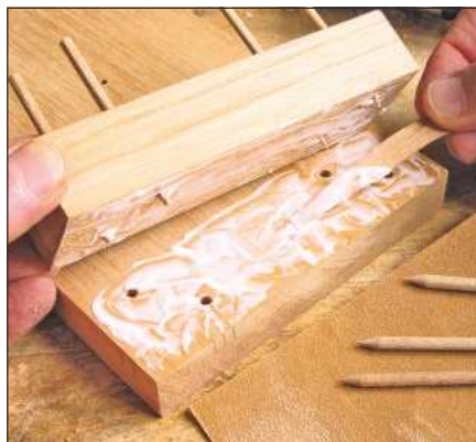
I assembled my bench hook using lots of glue and an assortment of kebab sticks
