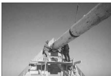
With one end in position, the other was carefully threaded into its cutout
