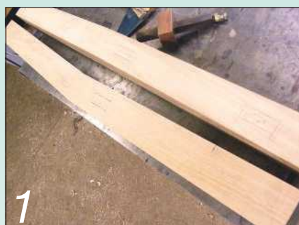
1 Mark the outline for both rear legs on the timbers and cut their profiles
