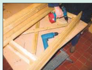
12 Add one or two cross braces if necessary to stop the structure from racking
