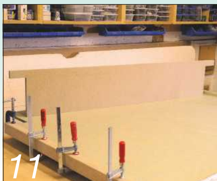
11 I fitted mdf mouldings round the headboard and cut a piece to fit across the bottom
