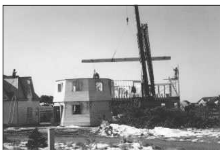
The log – soon to be The Great Beam – was carefully craned into the sky...
