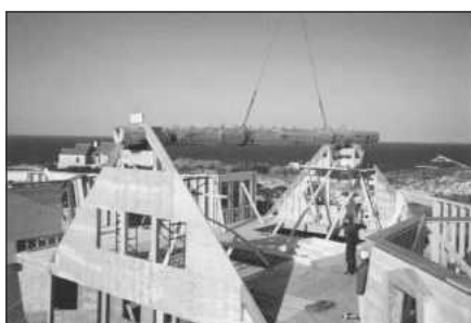
Each end had to be fitted into a circular cutout in the timber-framed gable
