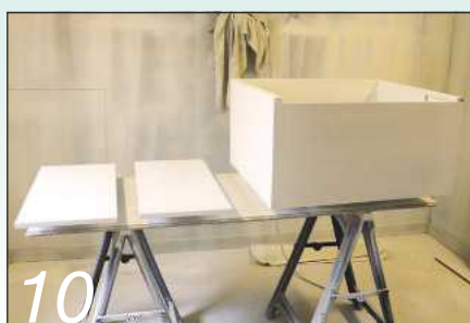
10 If you don't have a spray room, you can use a small foam roller to apply the paint
