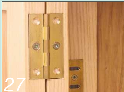
27 Initially fit the hinges with just a single screw
